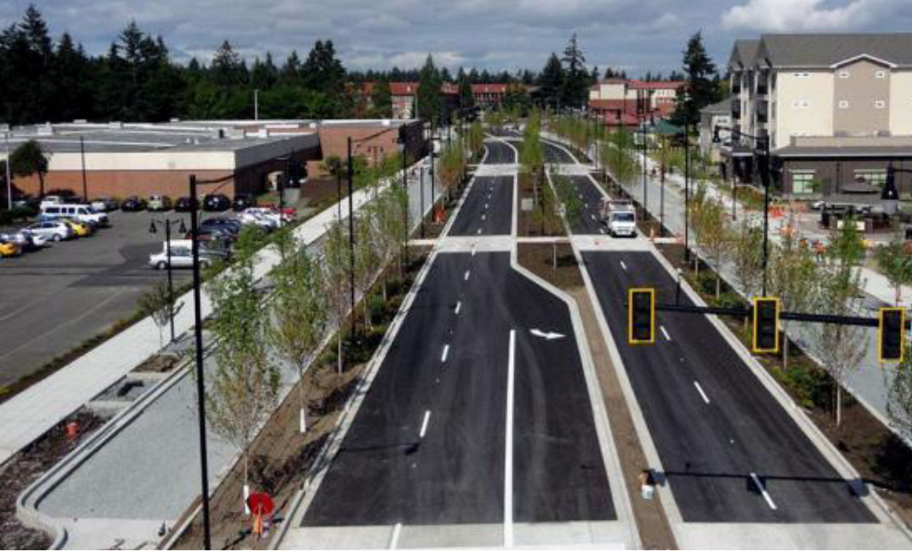
Figure 43: A raised median can calm traffic and provide a safe place for people crossing to access transit.
