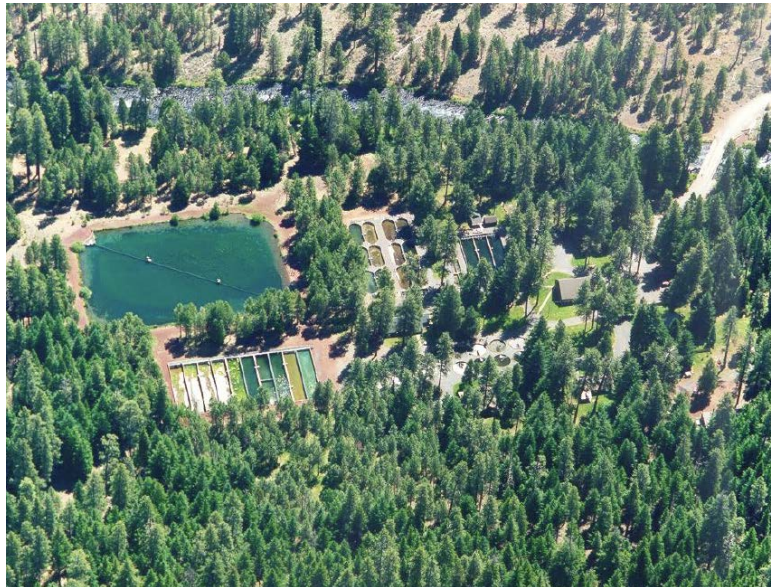
Figure 3.19. Wizard Falls Hatchery aerial photo, 1997. Courtesy ODFW, Wizard Fall Hatchery, Program Management Plan,” 2018, www.dfw.state.or.us
