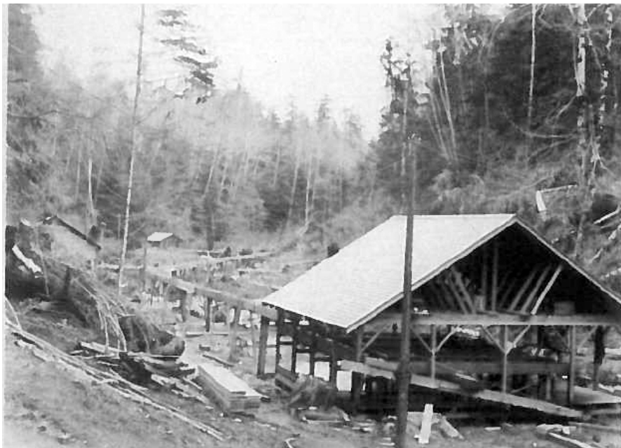
Figure 2.6. Unidentified salmon hatchery building and wood flume c. 1910. Courtesy Oregon Historical Society Research Library, OrHi 3499, Lot 790, Box 19, Folder 14.
