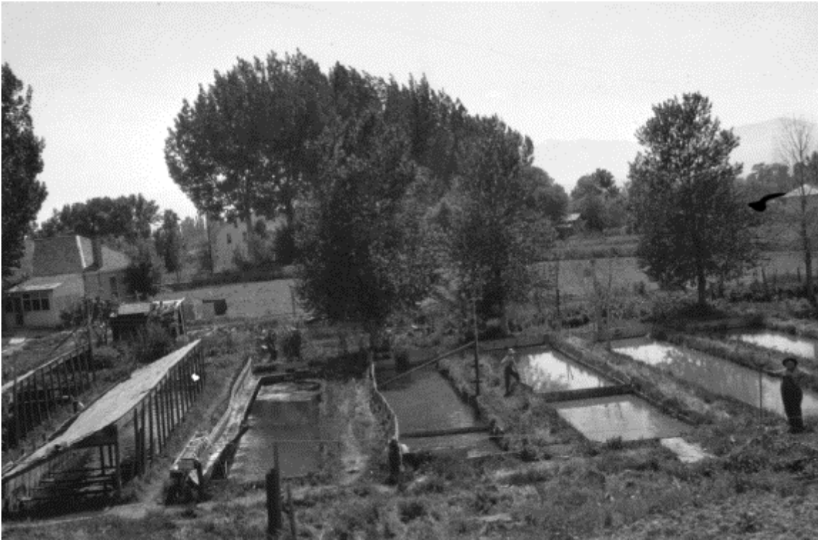
Figure 2.7. Wood-lined, earthen rearing ponds at Millcreek Hatchery, Salt Lake County, Utah c. 1890. Courtesy George M. Ottinger photograph collection, P0123, Special Collections and Archives, University of Utah, J. Willard Marriott Library, Salt Lake City, Utah.
