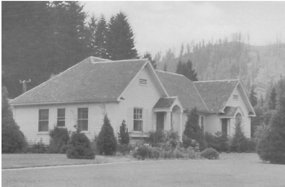
Figure 3.3. "Foreman's Residence, Alsea Trout Hatchery" c. 1941. Courtesy Oregon Historical Society Research Library, OrHi 3499, Lot 790, Box 11, Folder 1.
