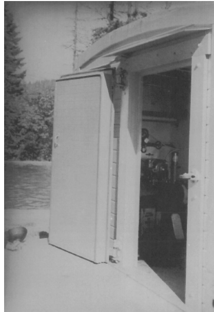
Figure 2.8. Cold storage building with insulated door c. 1935. Courtesy Oregon Historical Society Research Library, OrHi 3499, Lot 790, Box 19, Folder 5.
