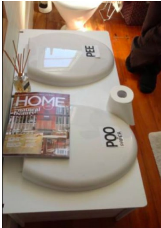
Figure 12: Christchurch No-Mix composting toilet design
