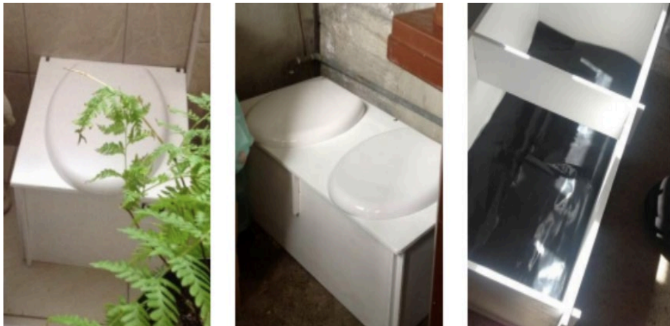
The flexibility of the emergency compost toilet. Left: Part of ‘split’ toilet installed in narrow space in a bathroom. Middle: Compost toilet located in an outside laundry. Right: A lined unit located in spare room of the house. Source: WREMO, 2012.
