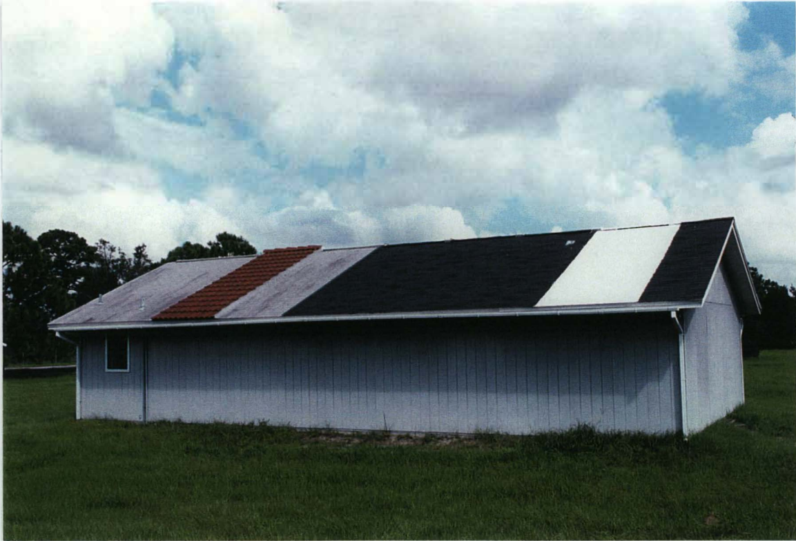
Figure 7-6 The FSEC Flexible Roof Facility
