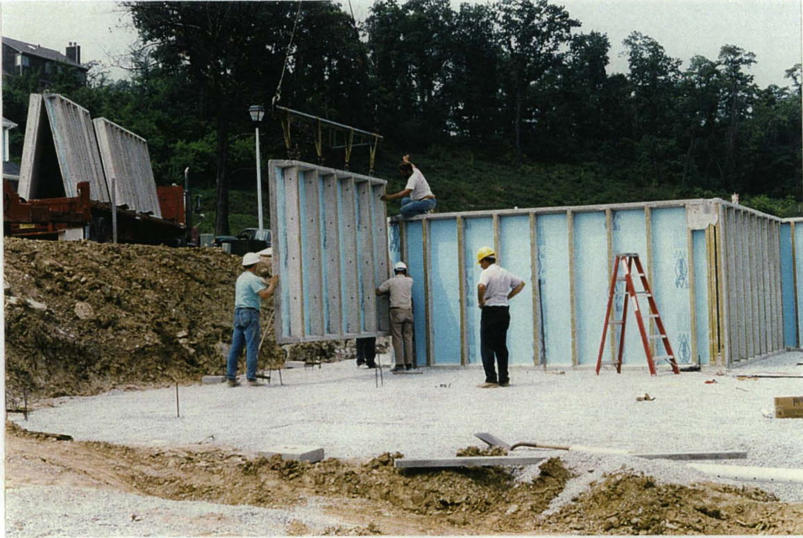
Figure 10-1 Superior Foundation Panel is Positioned
