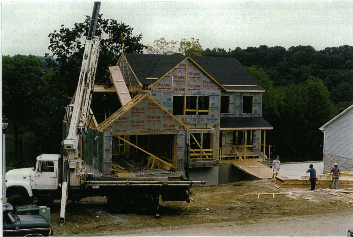
Figure 10-2 MIT Roof Panel is Hoisted in Place
