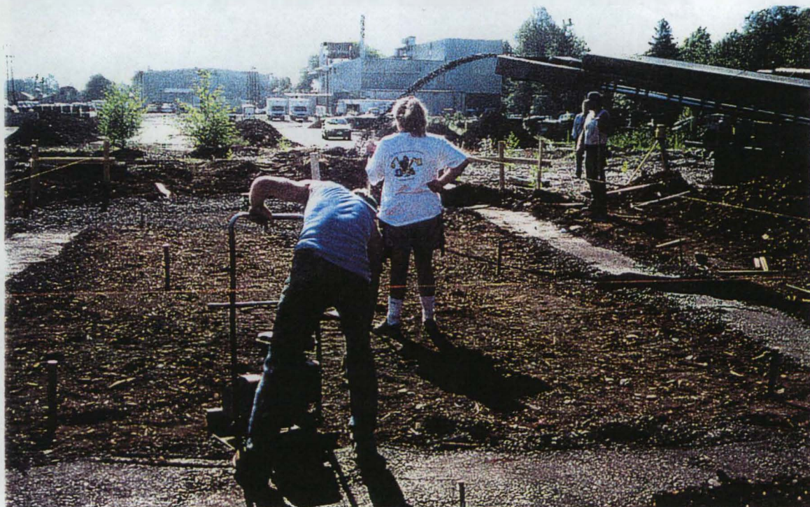
Figure 3-5, Placing and Compacting the Gravel Footer
