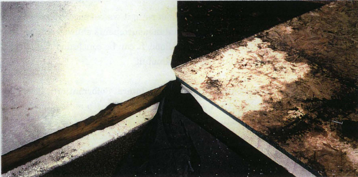
Figure 6-1, Chemical Deformation of Insulation and Panel Foam
