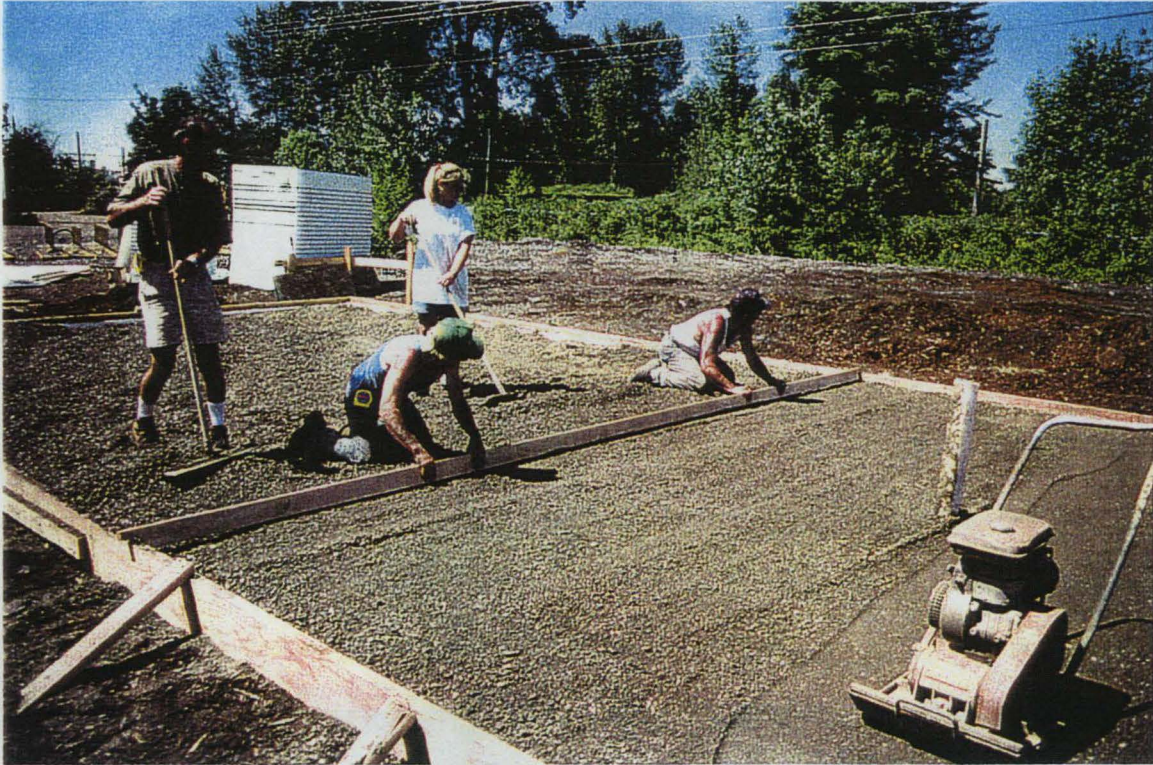
Figure 3-7, Leveling and Compacting the Gravel Fill
