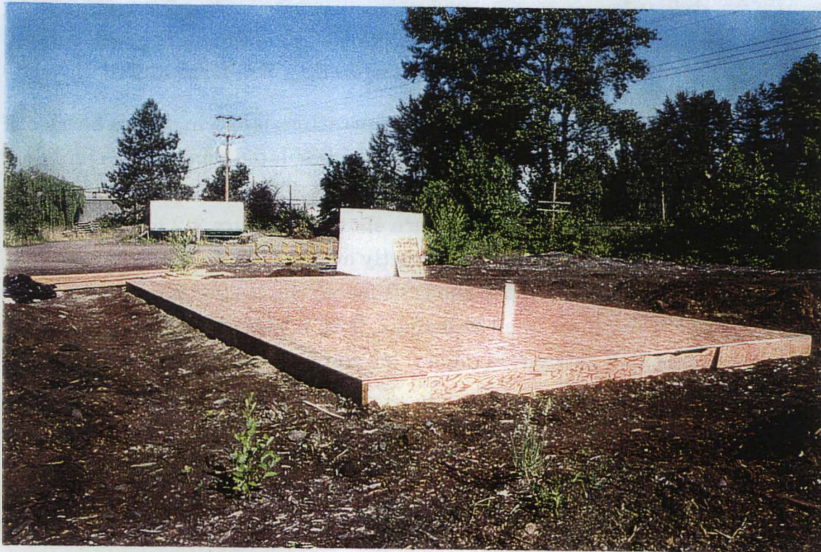
Figure 3-9, Completed On-Grade Insulated Panel Test Floor
