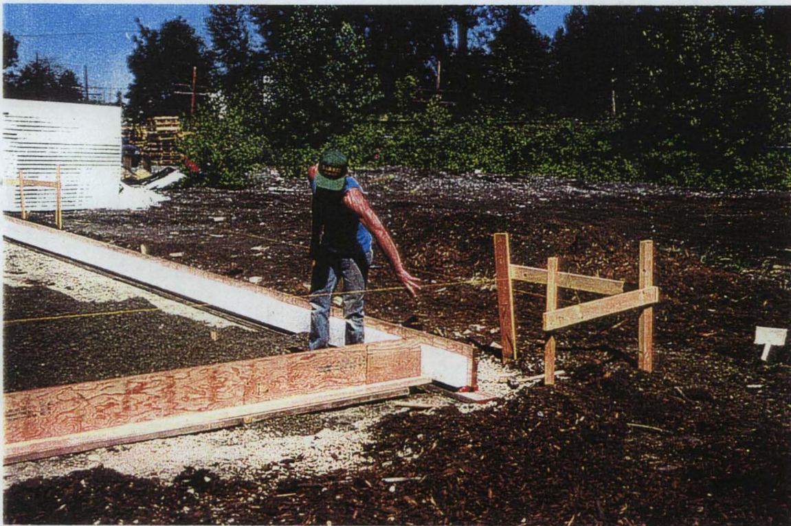
Figure 3-6, Installing the LVL Perimeter Beam
