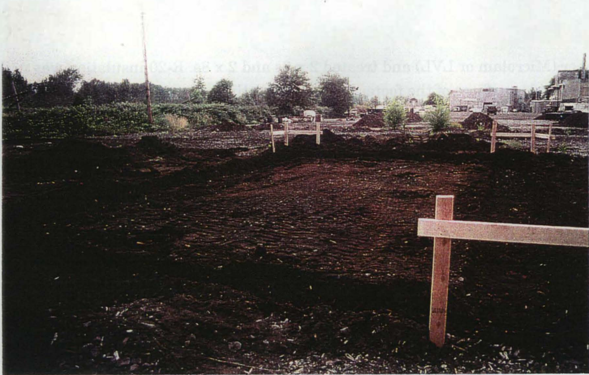
Figure 3-4, Excavation of the Footer Trench
