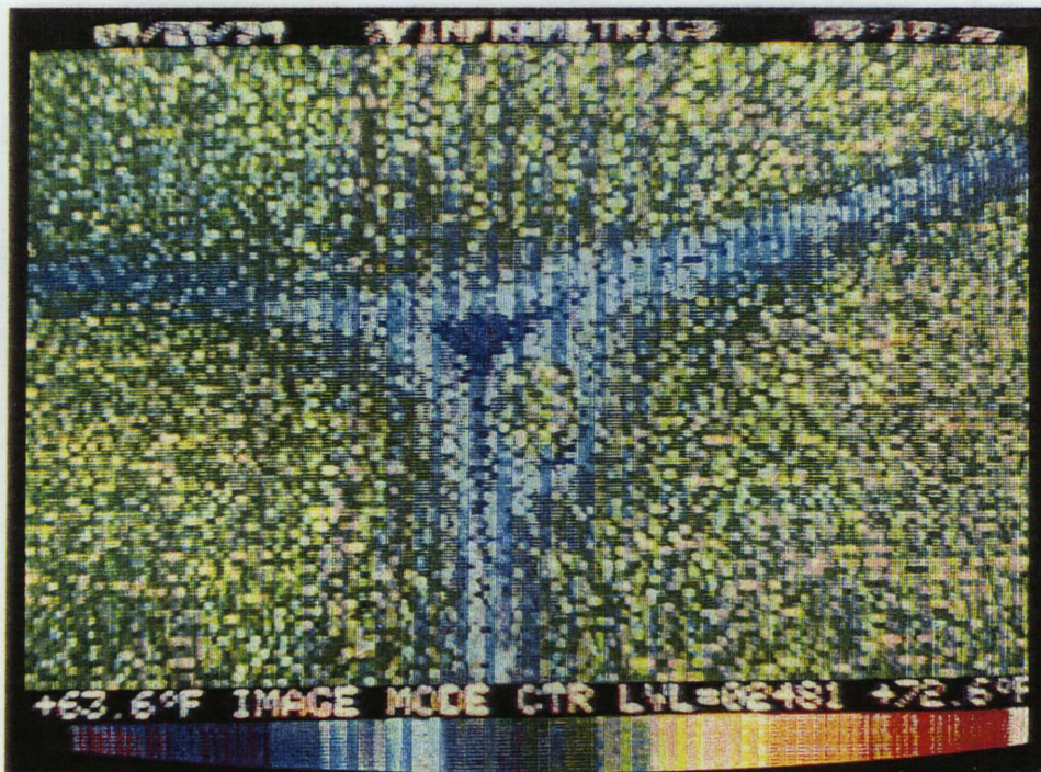
Figure 4-10 Heat Loss at Intersection of Panels and 2nd Floor Framing, Heat Loss through Fresh Air Vent also Visible
