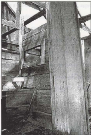
Figure 47. Horse Barn, Detail Showing the Divider Wall Between Stalls.
