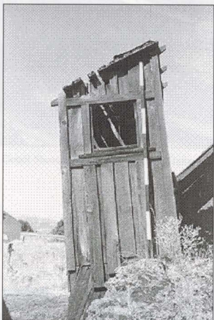
Figure 36. Outhouse, East Elevation.
