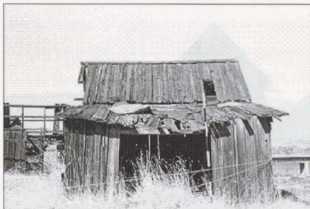
Figure 24. Visitor's House, East Elevation, Showing the Ridge Cap.
