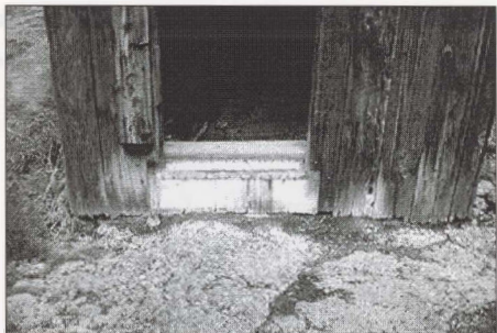
Figure 32. Chicken Coop, Detail Showing the Raised Entry and Metal Flashing.
