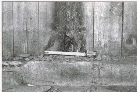
Figure 63. Chicken Coop, Interior, Fire Damage on the Rear Wall.
