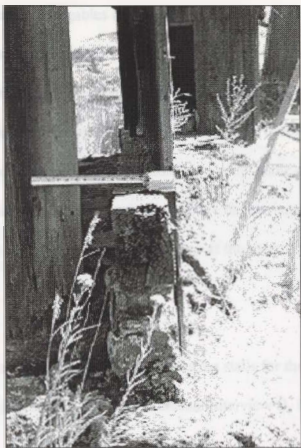
Figure 44. Horse Barn, Southwest Corner, Detail Showing Exposed End of the Sill/Foundation.
