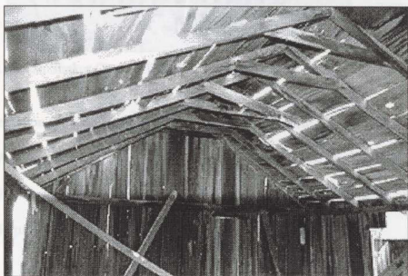
Figure 55. Indian Shaker Church, Detail of the Roof Structure.
