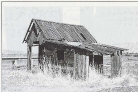
Figure 19. Visitor's House from the Southeast.
