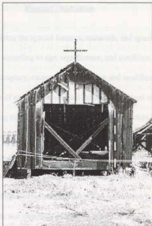
Figure 59. Indian Shaker Church, South Elevation, Opening for the Altar Bay.
