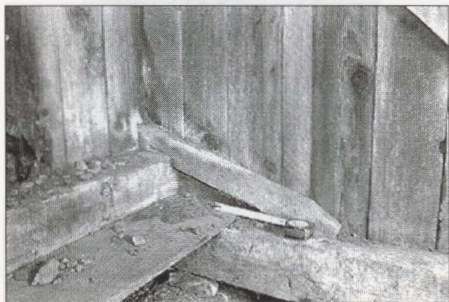
Figure 29. Chicken Coop, Interior, View of Stacked Sills in the Southeast Corner.
