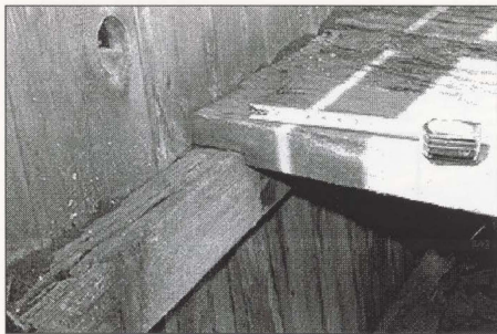
Figure 40. Barn (Small), Detail Showing Floor in the Upper Level.
