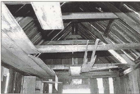
Figure 27. Visitor's House, Interior, Hung Ceiling in the Gable Portion.
