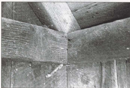
Figure 50. Storage Shed, Detail Showing End Lap Joint of the Top Plate.
