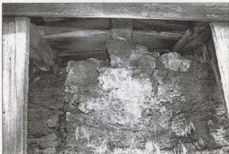
Figure 35 Outhouse. Detail Showing Underside of the Sill/Floor Structure.
