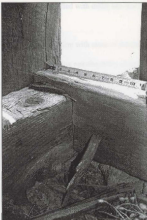
Figure 67. Horse Barn, Detail Showing the Sill in the Southwest Corner.
