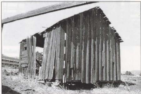
Figure 56. Indian Shaker Church. Detail of the North Gable End.
