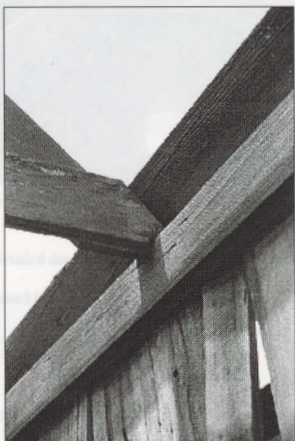
Figure 17. Detail Showing Character-Defining Feature: Connection at Eave Between Rafter, Top Plate, and Wall Boards.
