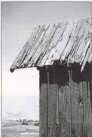
Figure 61. Chicken Coop, Detail of Roof at the Southwest Corner.
