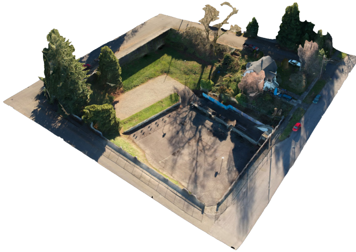
//Figure 3.2 Photogrammetric model from drone photography.
