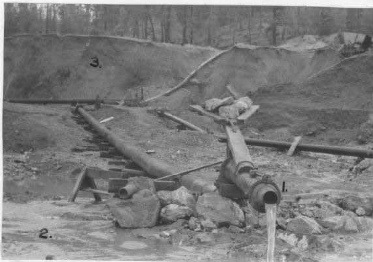
Figure 25. Speaker Placer. Giant (1) and pipe lie atop bedrock (2). Water pressure for the giant is achieved by dropping the water from a ditch located above the bank of valley alluvium (3).
