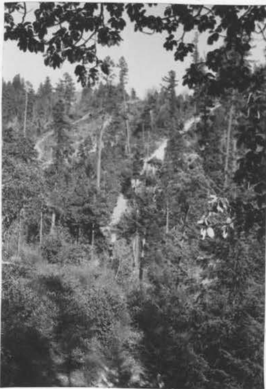
Figure 59. Skid roads leading out of an area where logging operations are being carried on. These narrow roads are built for tractor skidding to avoid "hang-ups."
