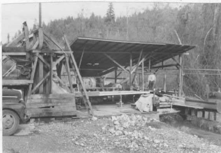
Figure 33. A small chrome mill approximately 10 miles southwest of Grants Pass on U.S. Highway 199. On the left is a small rock crusher and under the shed on the right is a concentrating table.
