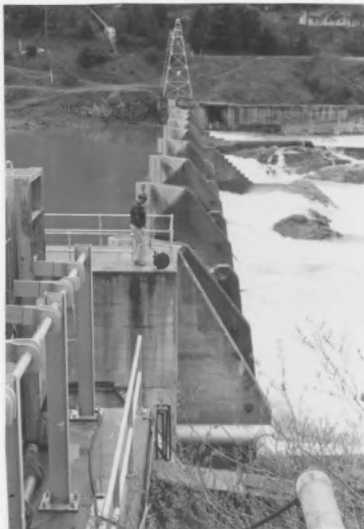
Figure 37. Savage Rapids Dam The dam is located on the Rogue River at the boundary of Josephine and Jackson Counties. The primary function of the dam is to provide water for irrigation. No electric power is generated.
