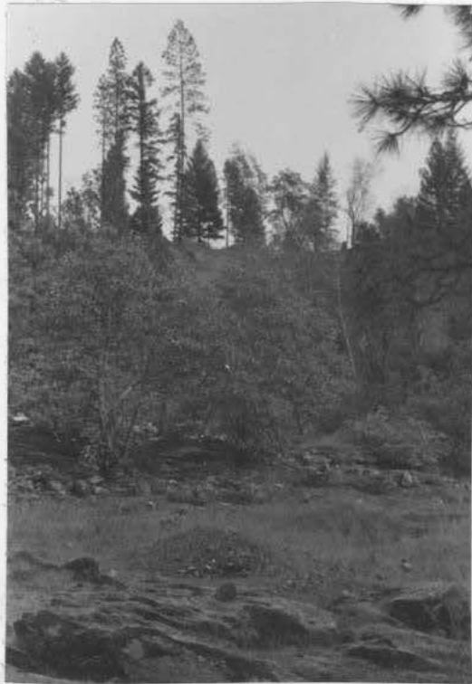
Figure 29. An Old Placer. The placer is located near Leland and is approximately fifty years old. Overgrowth of pine and manzanita partially hides the original bank-cut. Bedrock and small tailing piles may be seen in the foreground.
