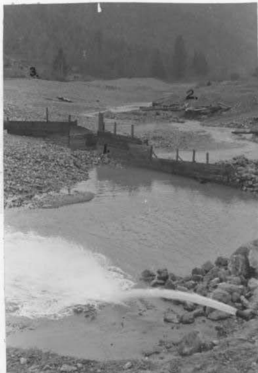
Figure 24. Speaker Placer. View looks west. The giant at the lower right is the same as appears in figure 23. Bank material is pushed over the sluice (1) and piles up as tailings (2). Wolf Creek (3) runs along the south side of the mine.
