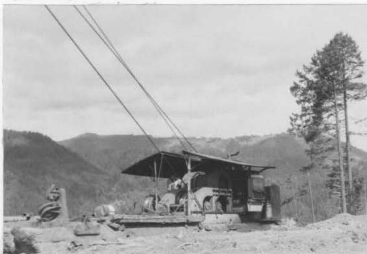
Figure 57. Large Scale Logging (high-lead yarding). Logs are yarded from the forest by cable and donkey engine (above) to a collection point near the spar pole (below). Here, using a logging arch (bottom left), the logs are loaded onto waiting trucks.
