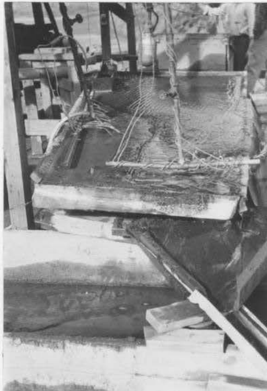
Figure 34. Chrome Concentrating Table. A small gasoline engine vibrates the table and the crushed raw ore is carried onto the table with water. Separation occurs on the lower right side of the table, the chrome being carried off the near right corner into a trough leading to a storage bin.
