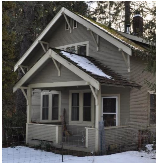
Image 22: Character Defining Features of #1004 include decorative brackets, horizontal siding, and original wood windows.
