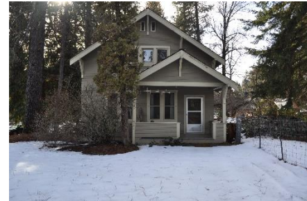
Image 12: Residence #1004, built in 1920. Historical view (top) and 2019 (bottom).
