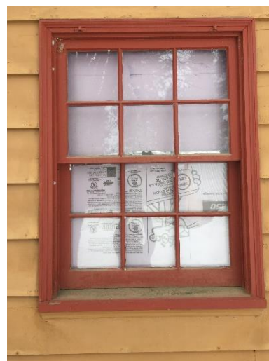
Image 44: Rigid Foam behind single-pane window in building #1018.
