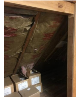
Image 41: Insulation in the attic of Building #2200
