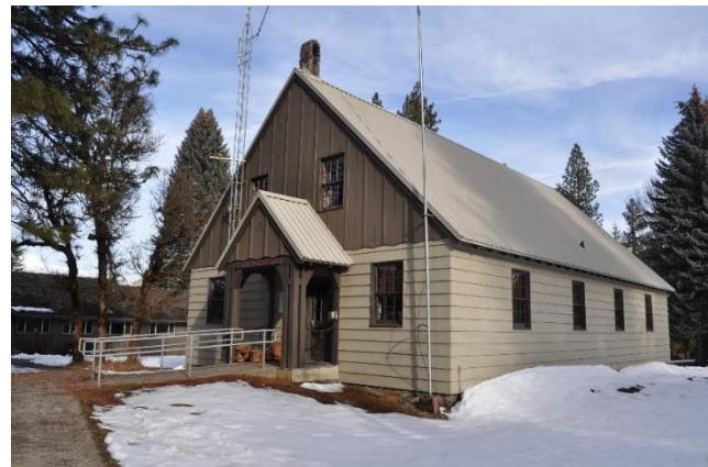
Image 28: Building #2200, Insulated and Weatherized Fire Warehouse now an Office
