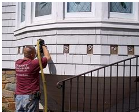
Image 42: Historic Shingles are Removed and then put back after insulation is blown into wall cavity. Source: NPS Preservation Brief 3.
