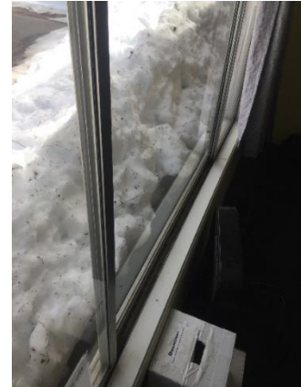
Image 53: Single Single-pane Storm Windows in #1019
