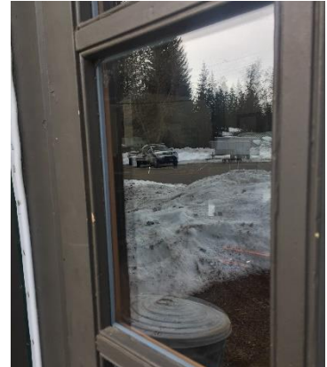
Image 50: DIY Double-pane replacement in original wood door frame done by Forest Service personnel
