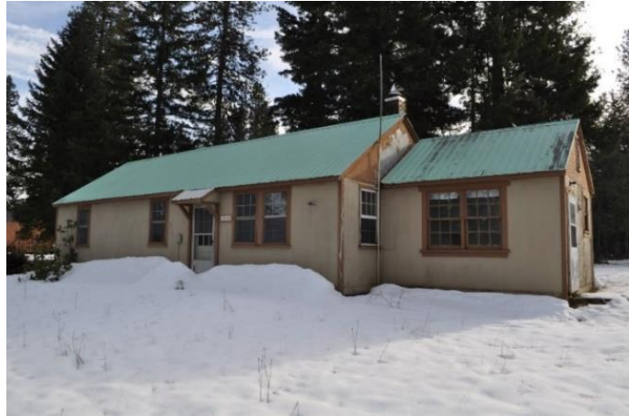
Image 18: Building #1003, a prefabricated building built in 1947.
