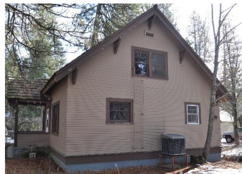
Image 34: Historic wood windows (bottom left) and replacement vinyl window (bottom right) shows negative impact of vinyl windows to historic character
