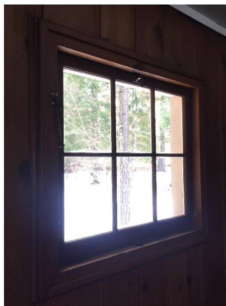
Image 45: Interior of Awning Windows in Residence #1300
