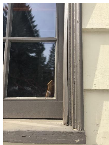
Image 35: Replacement vinyl frame around wood window on Building #2200 at Trout Lake – warping after just 10 years in service.
