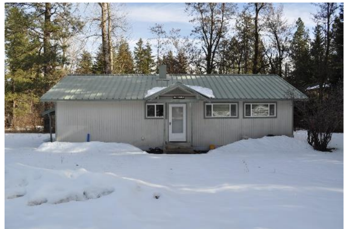
Image 25: Barracks Building #1307 in 1966, top (Image source: Beyond Rustic ) and 2019, bottom. Note replacement standing seam metal roof and vinyl windows
