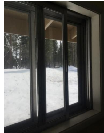
Image 54: Operable Single-Pane Prime and Storm Windows in #1019
