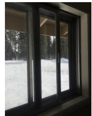
Image 54: Operable Single-Pane Prime and Storm Windows in #1019
