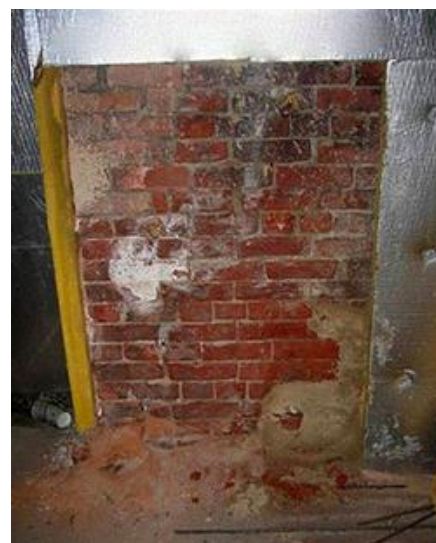
Image 31: Damage to Masonry from over insulating. Image: NPS Preservation Brief 3.
