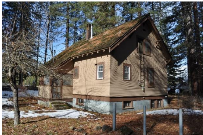
Image 23: Replacement vinyl windows on Residence #1001
