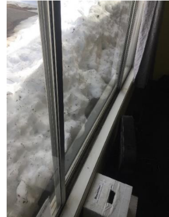
Image 53: Single Single-pane Storm Windows in #1019
