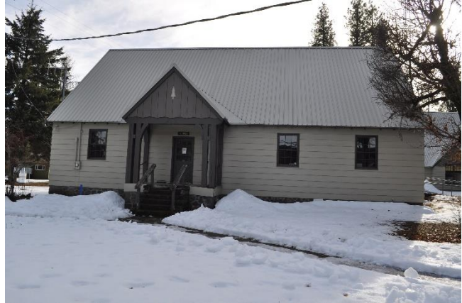
Image 8: The Fire Warehouse (#2200), built in 1936 by the Civilian Conservation Corps.
