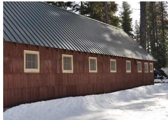
Image 24: Building #1300 at Trout Lake, built in 1936 now has a replacement standing-seam metal roof.
