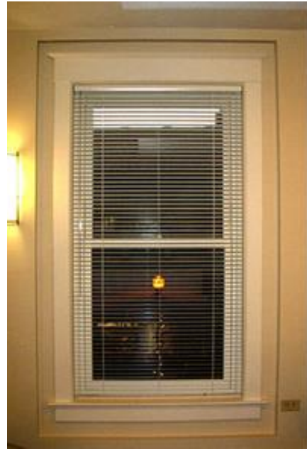
Image 32: New interior walls negatively impacted the historic character of this building. Image: NPS Preservation Brief 3.
