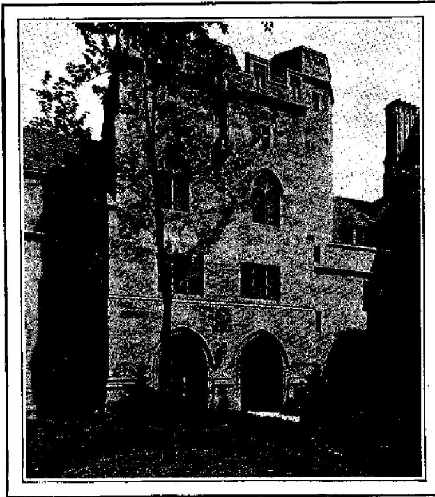
Harkness Memorial Residence Halls, Yale University, James Gamble Rogers, Architect. Detail view in one of the Courts showing "Rippleface" finish Indiana Limestone
