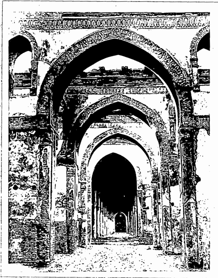
Fig. 11. Mosque Ibn-Tulūn Cairo IX century Exterior
