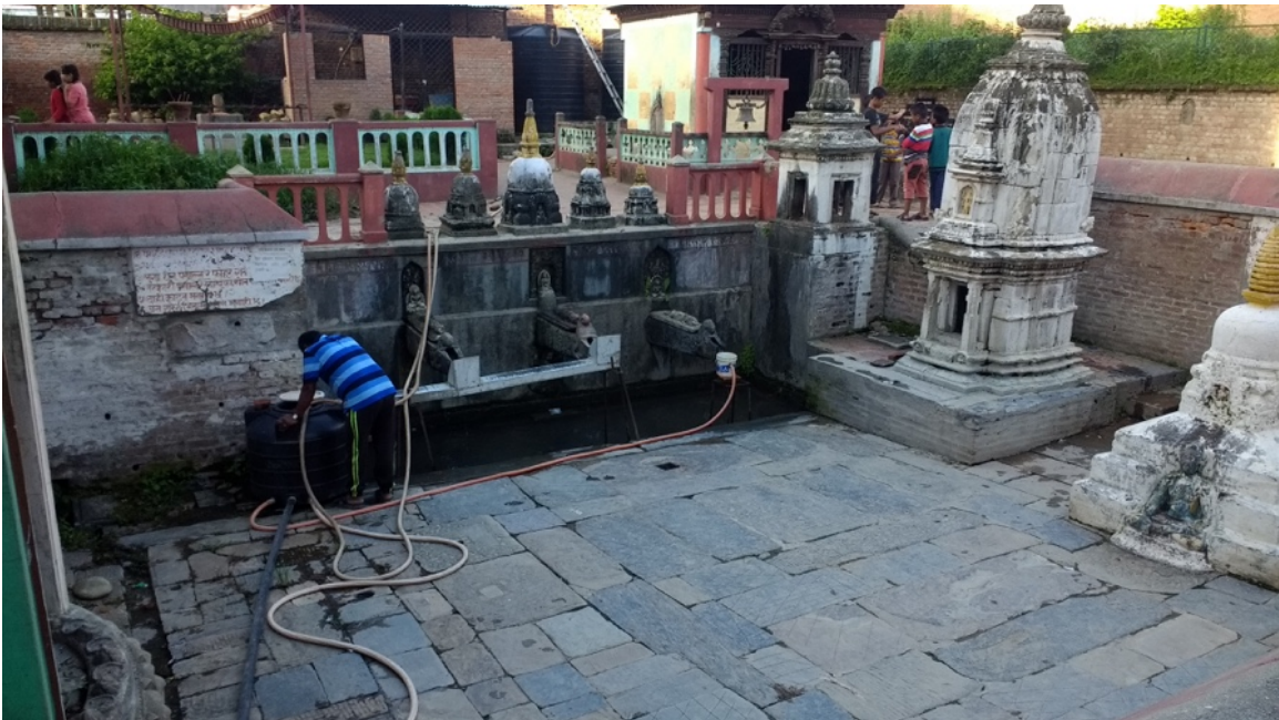
Figure 38. Aalko hiti's water collection system and recharge area.
