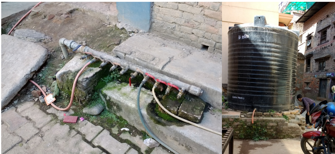
Figure 39. Samrat’s water access points: piped stone spout water in the wet season and tanker water in the dry season
