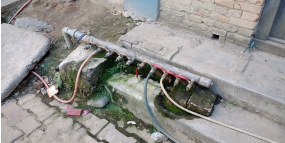
Figure 21. Samrat's access point to Aalko Hiti's micro grid system that pumps water from an ancient stone spout. Samrat's story-map: https://arcg.is/01LSGf
