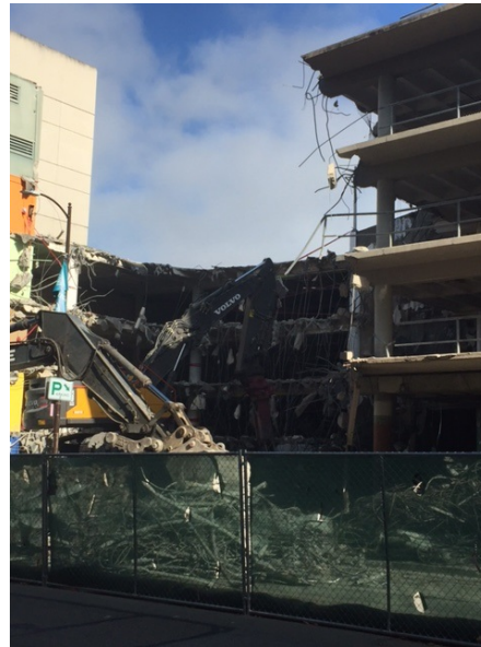
Further demolition of all levels
