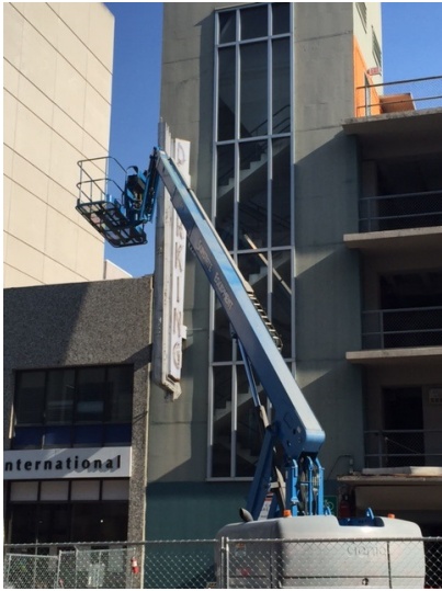
Dismantling of "parking" sign
