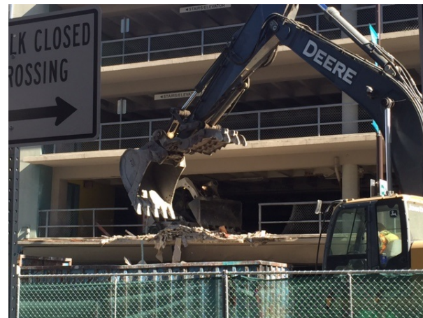
Second floor office demolition
