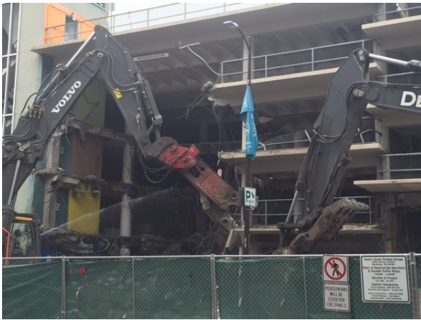
Demolition of Levels 1-3
