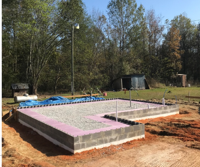
Fig 5. Elevated slab detail (NTS) and construction photo. Photo by Emily McGlohn
