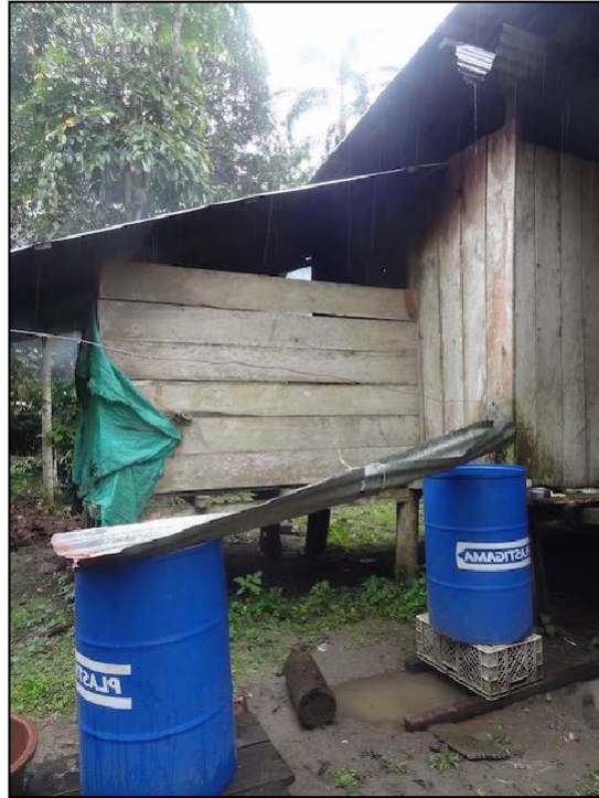
Fig. 2. Rain water collection system using tin roofs
