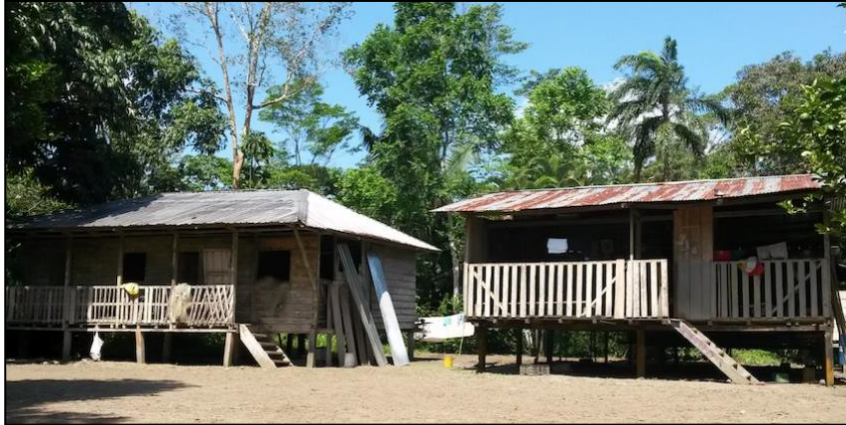
Fig. 6. Replacement of traditional roofs with tin ones at family homes
