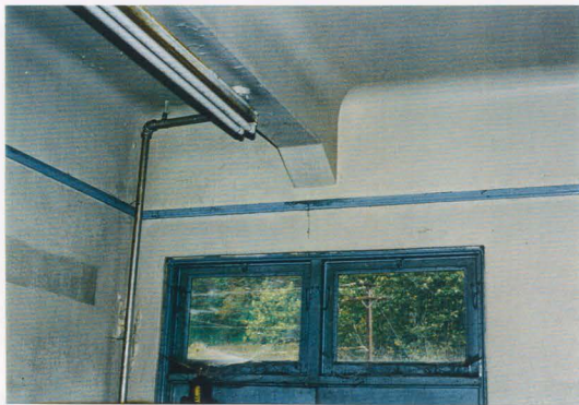
Detail at Interior of Front Door
