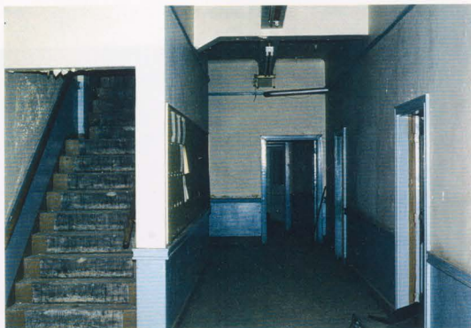
Entry Hallway - First Floor
