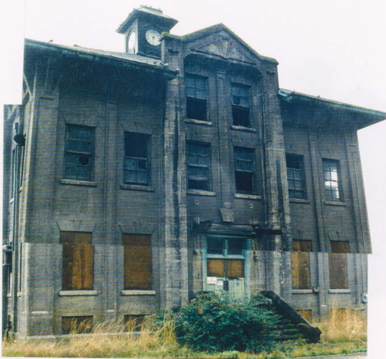
Front of building
