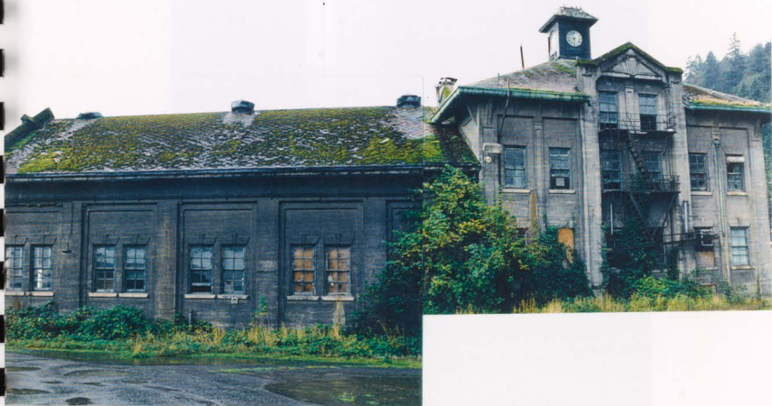
North side of building
