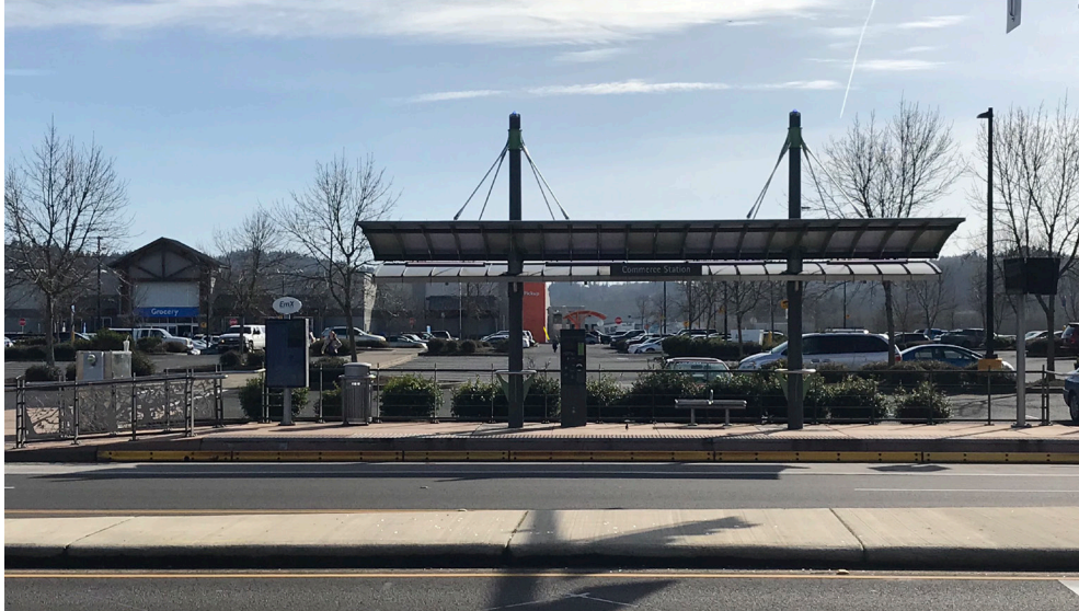
FIG. 2 Commerce Station: View of the project site from the north.
