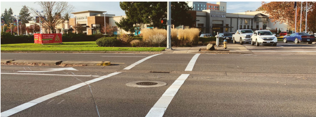
FIG. 1-1 An extended crosswalk over five lanes of traffic on Coburg Road near the Oakway Center.
