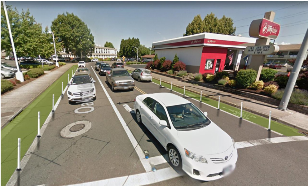
FIG. 2-4 Bollard-protected bike lanes on each side of Oakmont Way.
