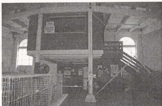
Fig. 30. Office in east end of poultry building, hiding transom and fanlight above door. Note staircase obscuring window; and small storage room under landing. Photograph by author, 2008.
