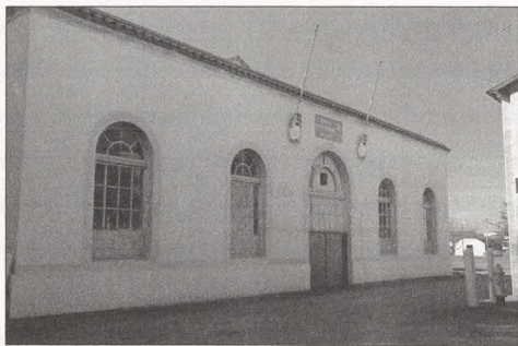
Fig. 17. East façade of poultry building showing walls with stucco finish and painted door and window trim. Photo by author, 2008.
