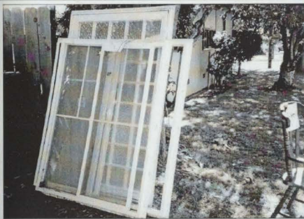
Vinyl framed "replacement" windows being removed after only four years of use. Twisted frames on a southwest exposure.
