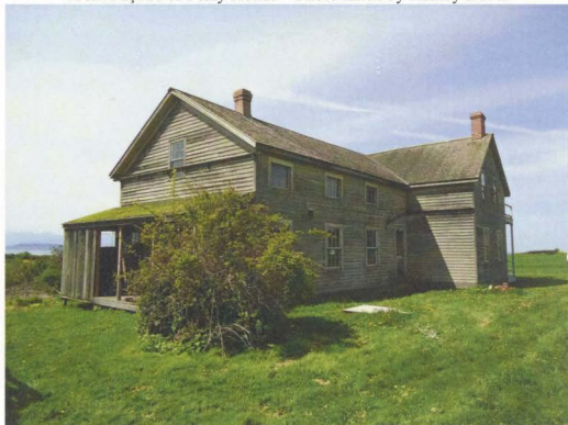
Back Façade of Ferry House – Photo taken by Ashley Davis
