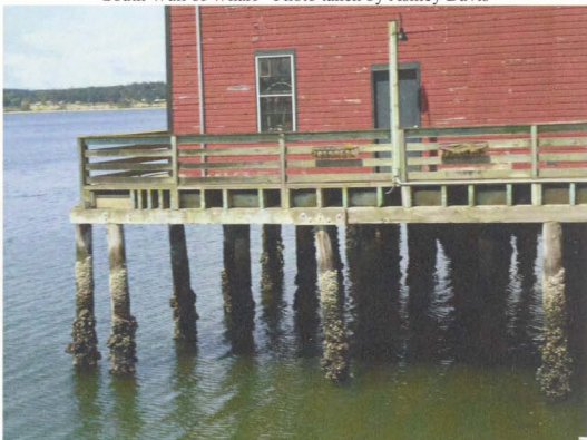
Foundation of Wharf - Photo taken by Ashley Davis
