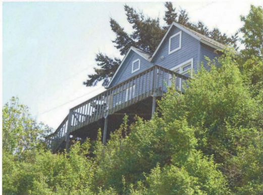
North Facade of Law Office - Photo taken by Ashley Davis
