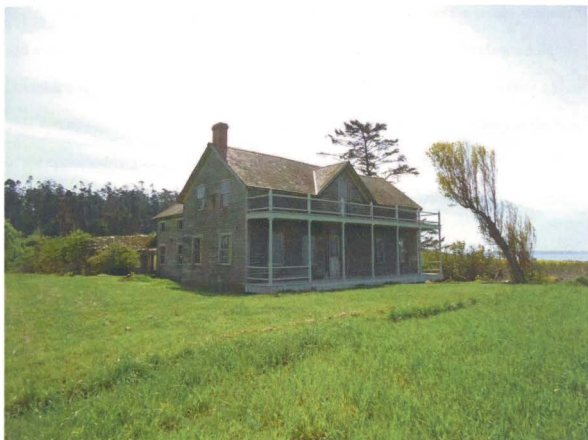
Figure 1.5 Ferry House front façade, looking southeast; taken by Ashley Davis.
