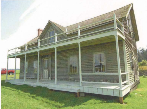
Front Façade of Ferry House – Photo taken by Ashley Davis
