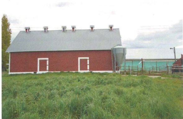
Figure 1.4 LeSourd Granary south façade, looking north; taken by Ashley Davis.
