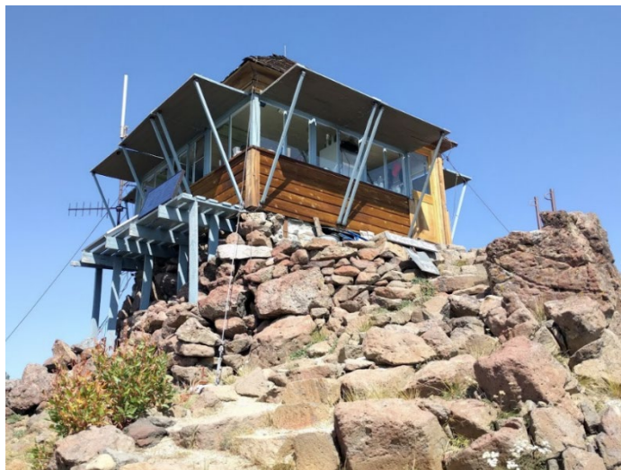
Southwest and southeast elevations and site
