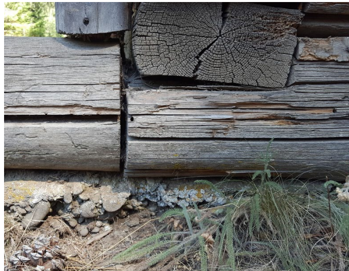
Foundation and sill construction
