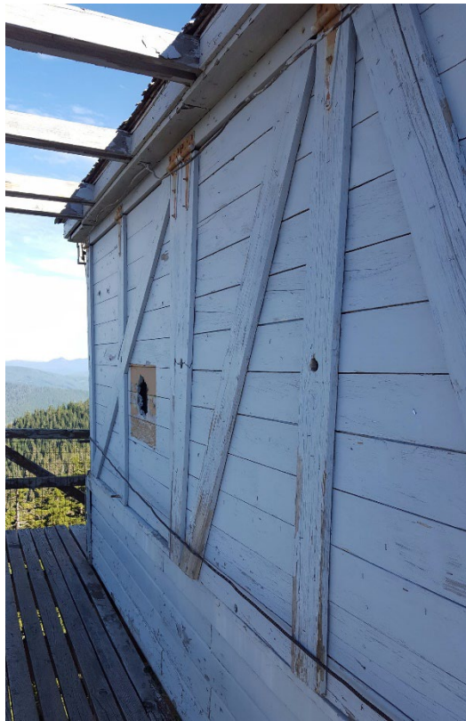
Typical condition, north elevation
