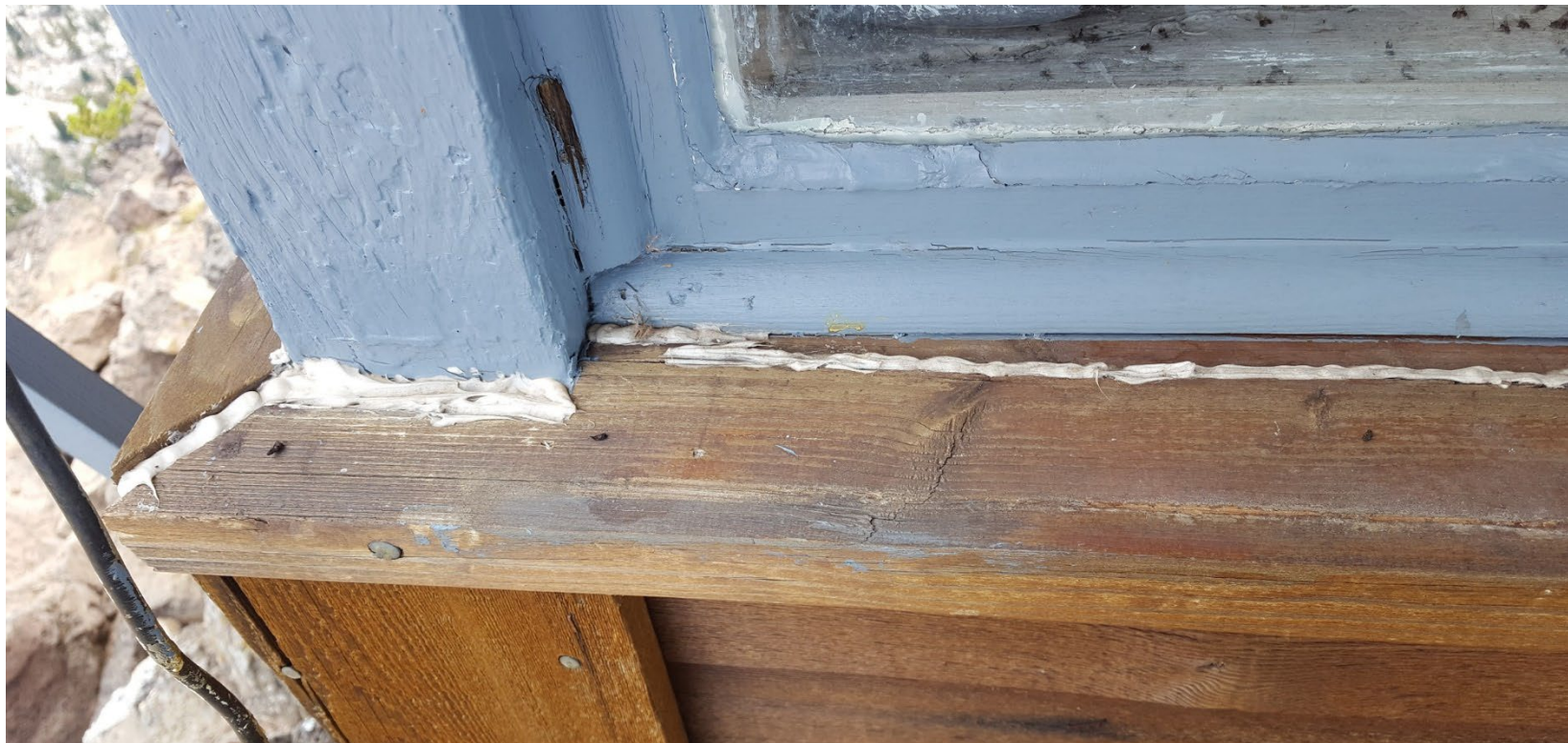
Typical condition of window sills, unpainted and caulked
