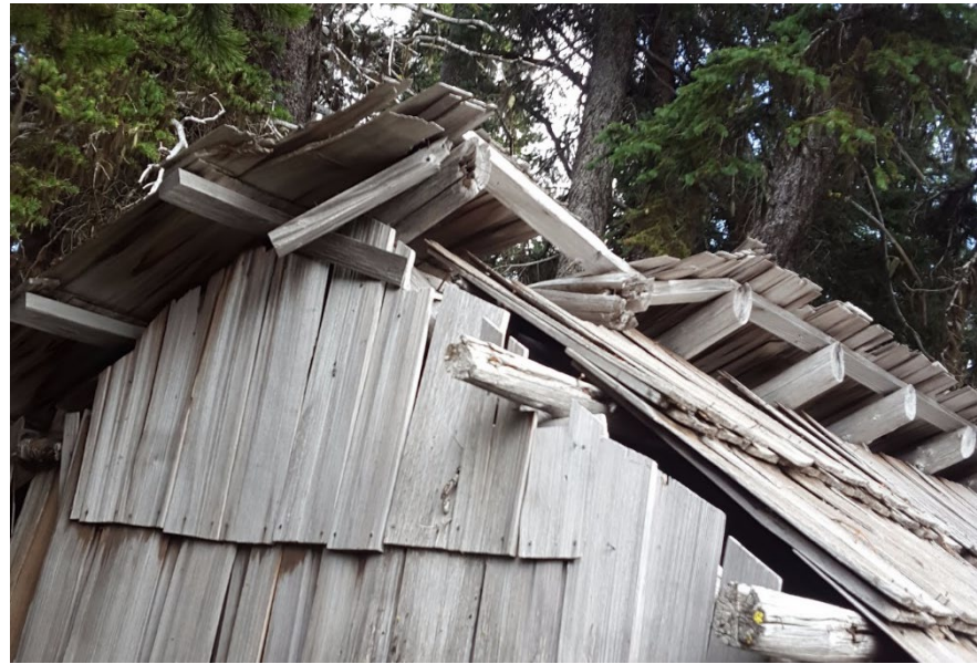
Roof construction and condition
