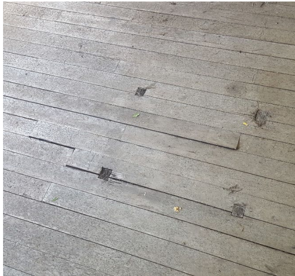
Typical construction and condition, absent Fire Finder
