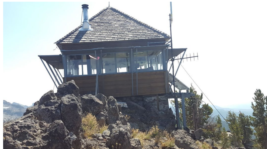
Northwest elevation and site
