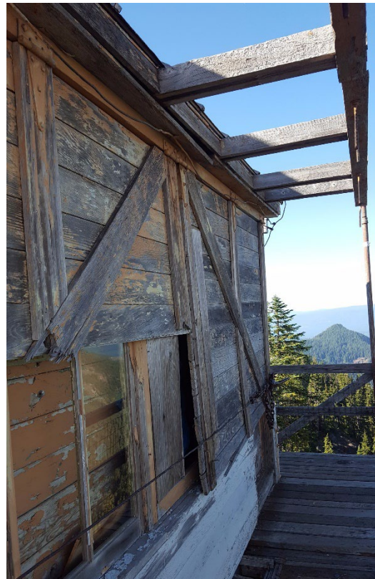
Typical condition, east elevation
