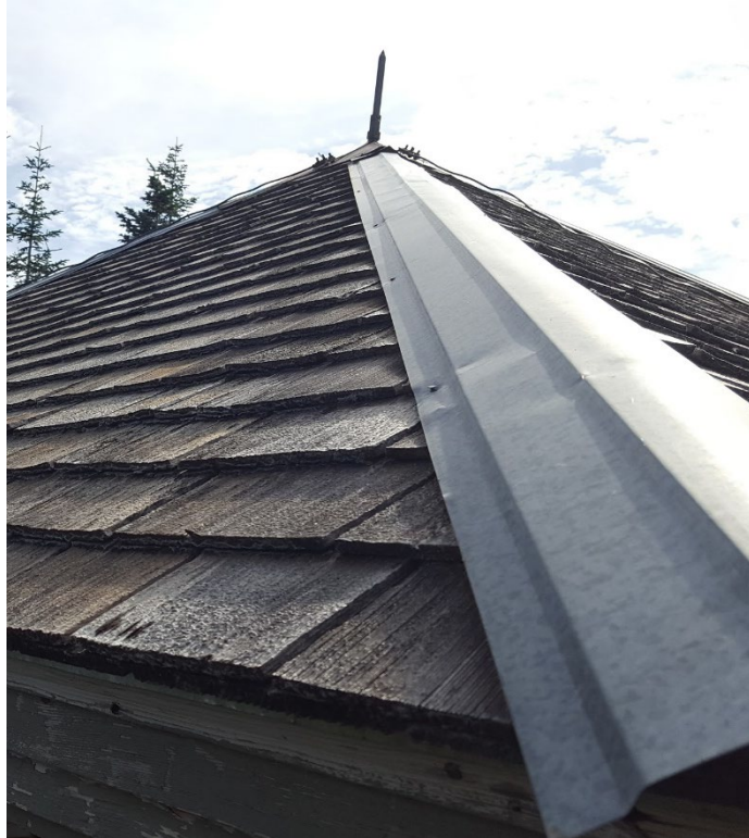
Typical condition, roof
