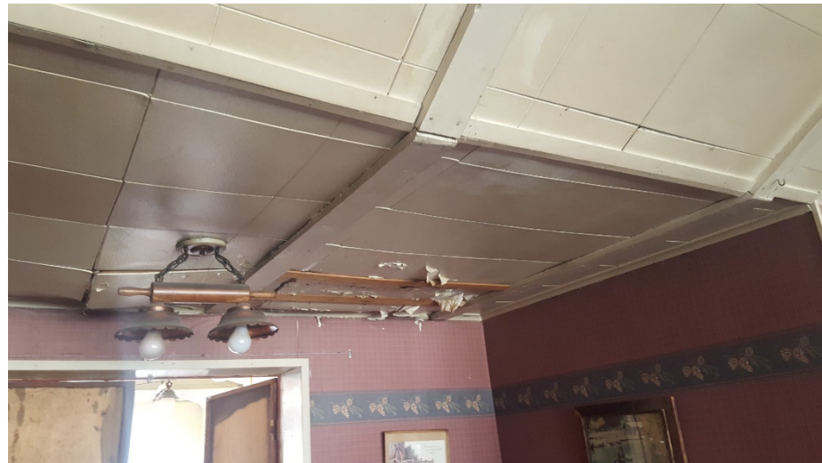
Dining hall ceiling condition
