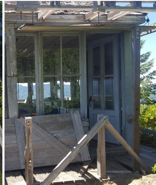
Altered northeast railing
