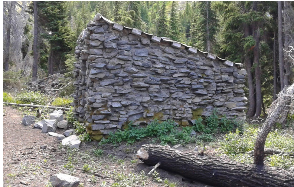
Site, north elevation
