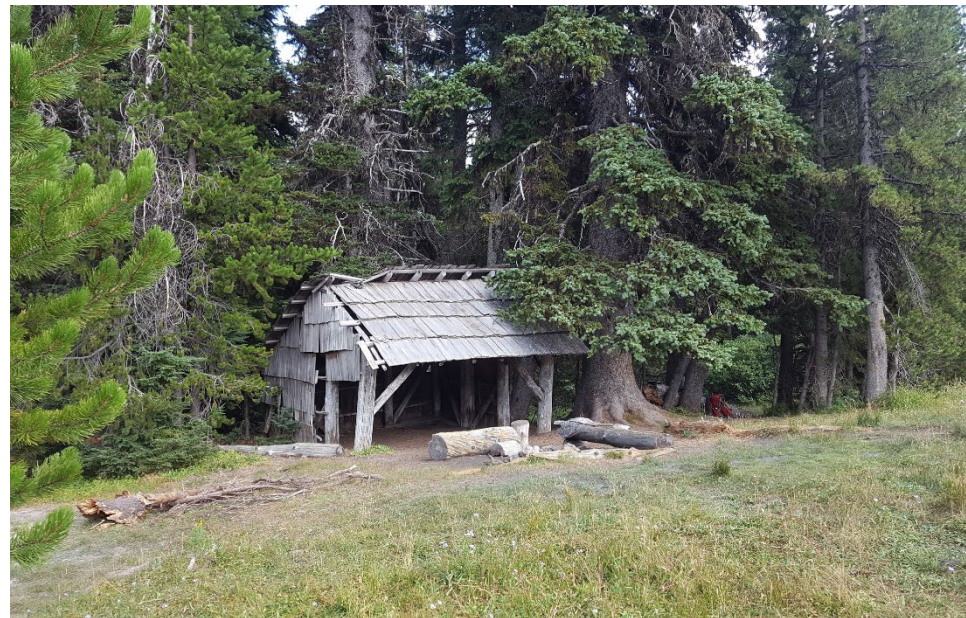
Site conditions, north and west elevations
