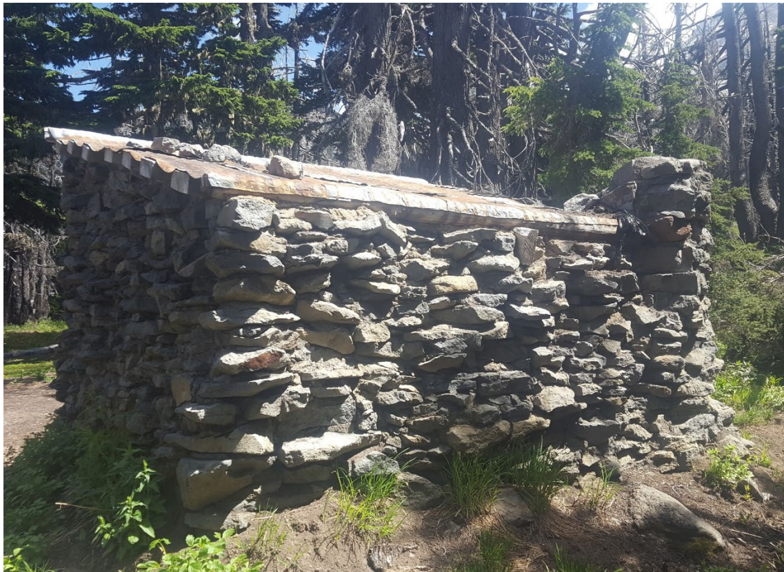
Rear elevation and chimney
