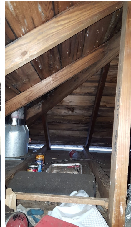
Typical condition, attic
