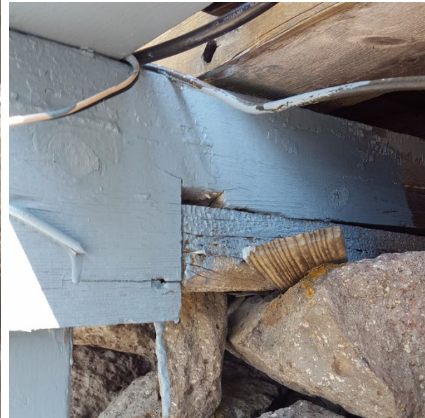
Typical rough construction of solar panel deck
