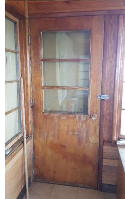
Door construction and condition
