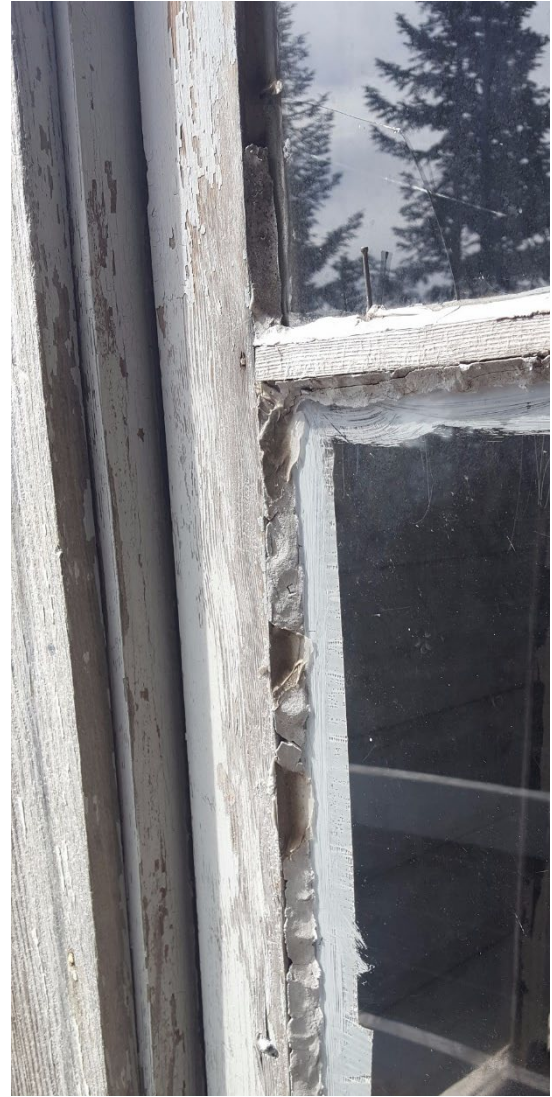
Typical condition, sash and glazing
