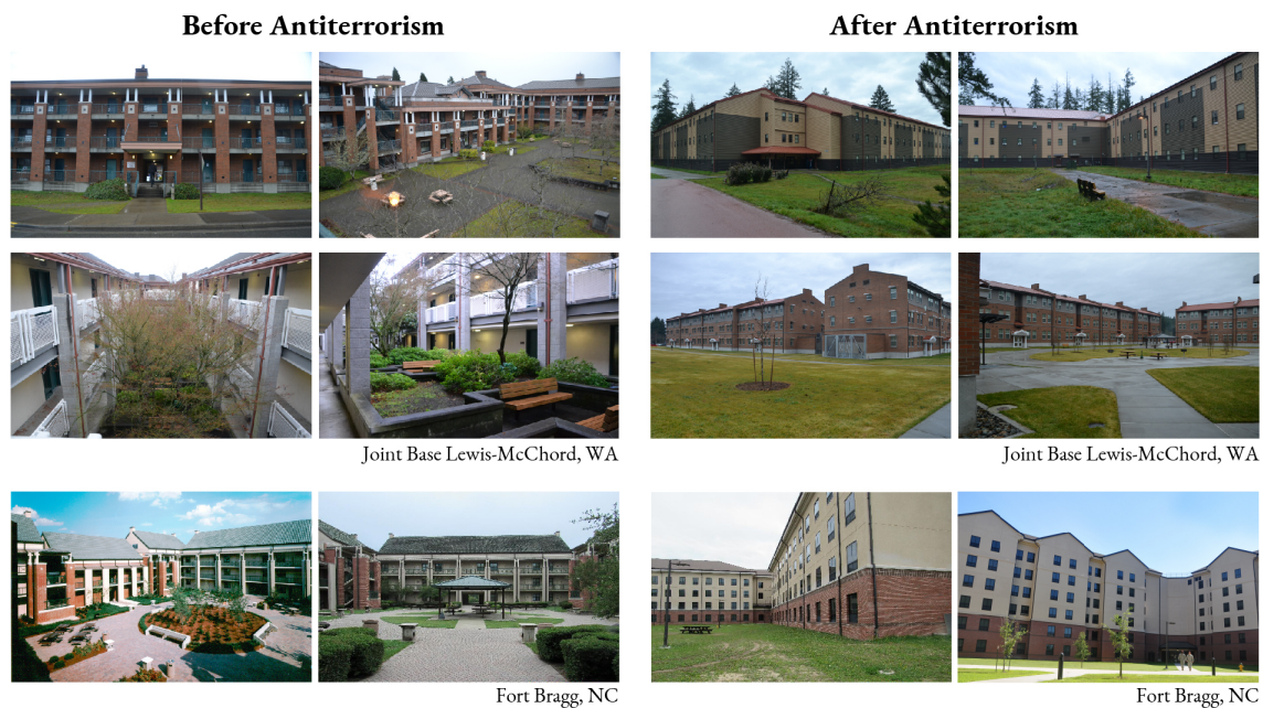
Figure 2.14. Barracks before and after antiterrorism. Fort Bragg images courtesy of Fort Bragg. JBLM images taken by the author.
