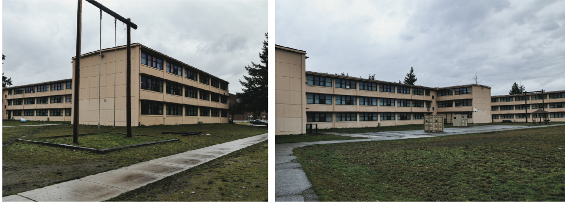
Figure 1.15. "H-style" barracks design at Joint Base Lewis-McChord. Images taken by the author.
