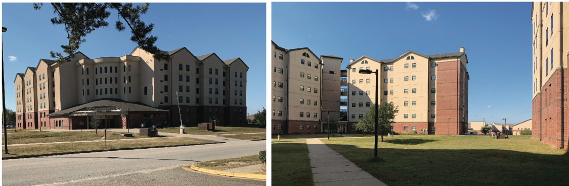
Figure 1.26. "One-plus-One, Enhanced" barracks at Fort Bragg. Images taken by the author.
