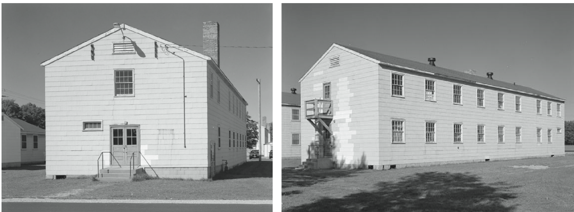
Figure 1.10. Quartermaster General 800-series standard design for mobilization barracks. Images from the Library of Congress Prints and Photographs Division, Washington, DC. Reproduction numbers HABS WIS,41-SPAR.V,1-A--6 (left) and HABS WIS,41-SPAR.V,1-A--4 (right).
