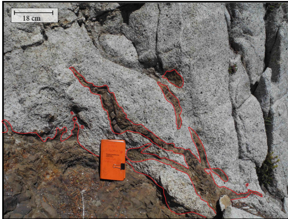
Figure A.5. An example of flame-like structure in a host-rock (granitoid) within the CJDS. This type of host-rock-dike interaction was only seen once in the 2016 and 2017 field seasons. The approximate location of this outcrop: 45.040663° N, 117.252655 ° W. Red lines are drawn around dike margins to highlight the degree of fragmentation.
