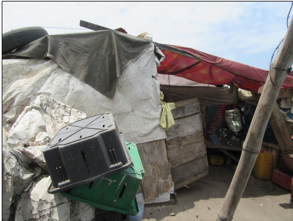
Figure 5.3. Faith's dwelling used recycled wood, fabric, and plastic tarps, held down by rocks, tires, and string (Source: Author, July 2019).
