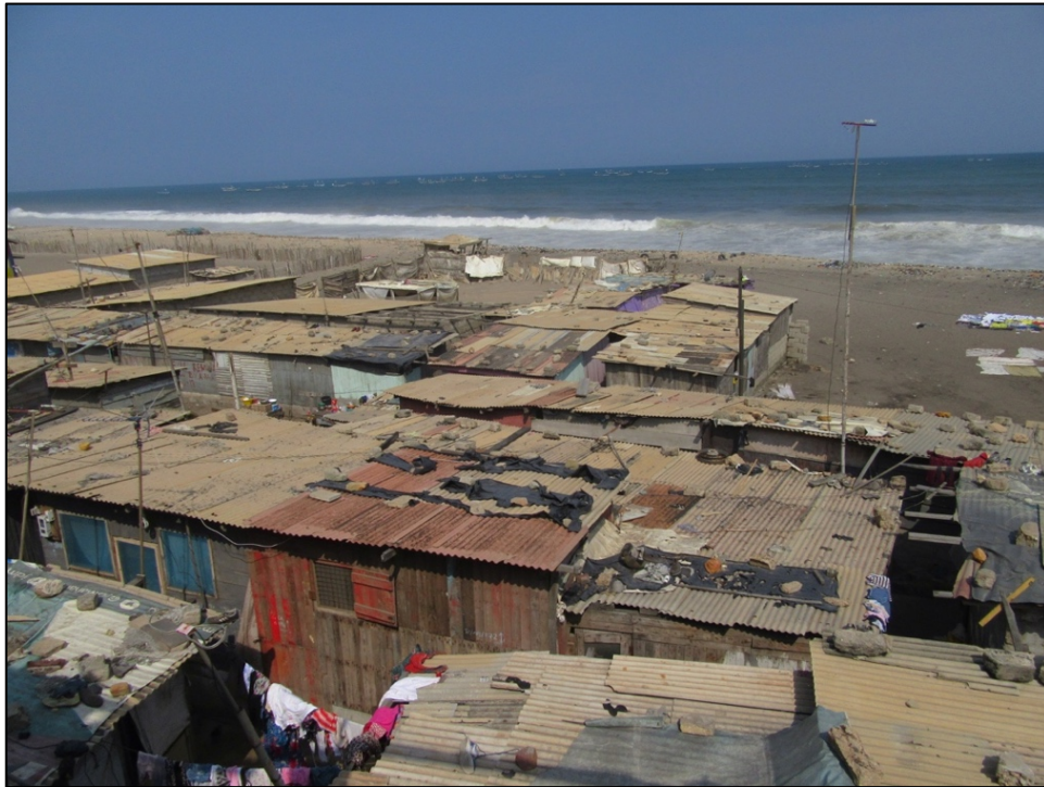
Figure 5.1. Corrugated iron sheets used for roofing, held down by rocks and other various heavy objects. These dwellings were located outside of the study site on the far side of the harbor, which has not been demolished since 2015 (Source: Author, July 2019).
