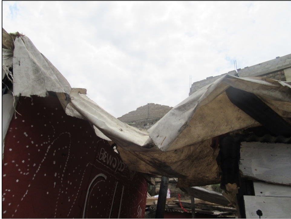
Figure 5.2. Plastic tarps were used as roofing in place of corrugated metal. Cheaper building materials like plastic and fabric were easily damaged by rain and sun, shown above as rips in these plastic tarps (Source: Author, July 2019).
