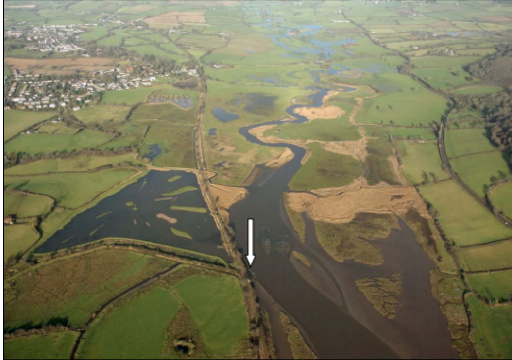
Figure 2: Tide gate location in watershed in Seaton, United Kingdom: Environment Agency UK.
