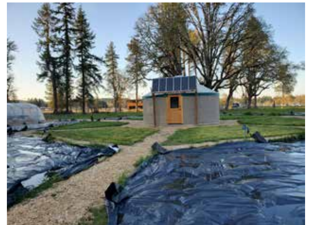
(Image by K. Parr) High school and community volunteers have been instrumental in installing the hard infrastructure. To further interest and community involvement, festivals are planned throughout the year. In the initial construction phase this summer seasonal favorites, such as strawberries, will be a delicious showcase of the school farm's potential.
