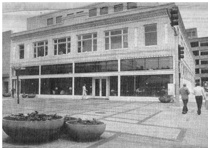
Figure 11.15. Images of the Ardel building in c. 1955 showing Nickles Shoe Store and Rudolph's Furs (top; sc. LCHM Catalog #GN1092) and the new Downtown Athletic Club building after Ardel's renovation (bottom; sc. Peggy Shekell as published in The Oregonian May 24, 1986).
