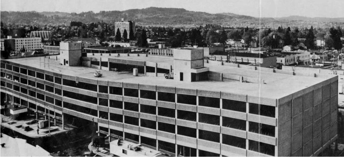
Figure 8.13. The 10 th and Oak "Overpark" garage was completed in 1969 (but it was not a part of CEP).
