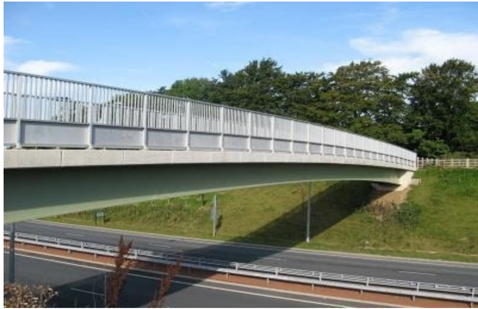
Figure 2.3: Steel Girder Pedestrian Bridge. Source: SteelConstruction.info
