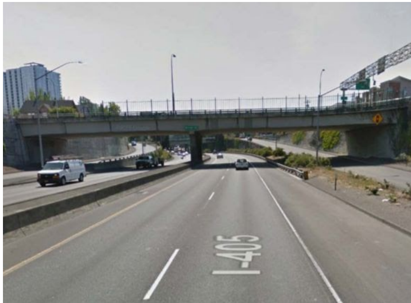
Figure 2.1: Typical Box Girder Bridge in Portland. Source: Google Maps
