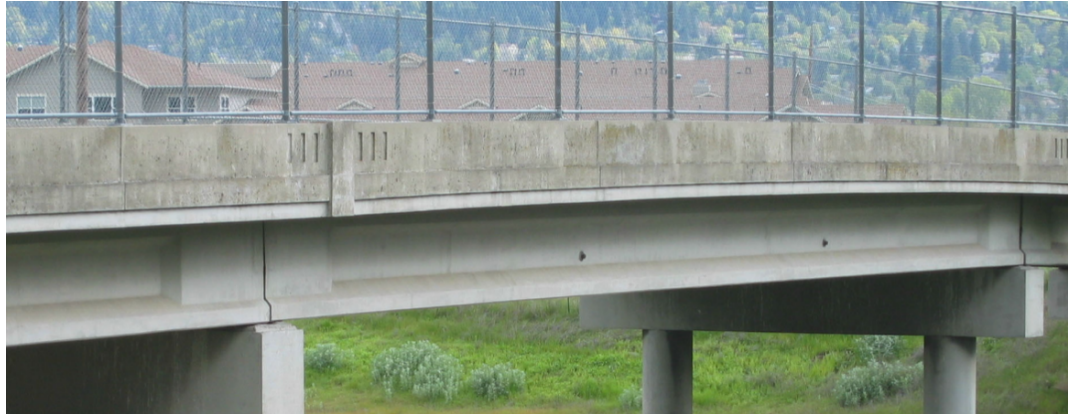
Figure 2.2: Oregon Precast Concrete Girder Bridge. Source: ODOT
