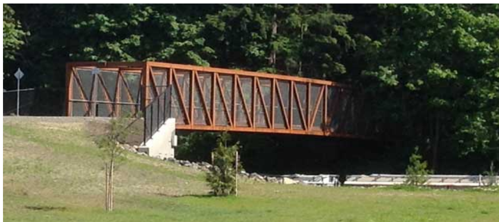
Figure 2.4: Steel Truss System. Source: Portland.gov
