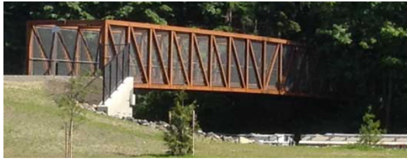
Figure 3.1: Truss Bridge. Source: Oregonlive.com
