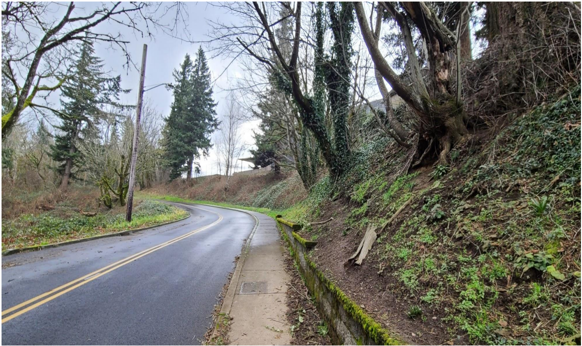
Figure 2: Photo taken near 6th St looking south west on SE Sandy Ave
