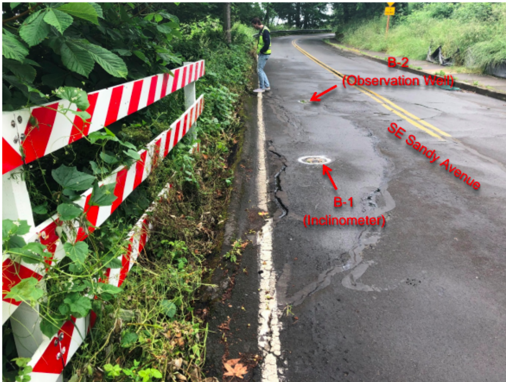
Figure 17: Area of Pavement distress along Sandy Ave near 4th St - Looking South (Shannon & Wilson, 2018).
