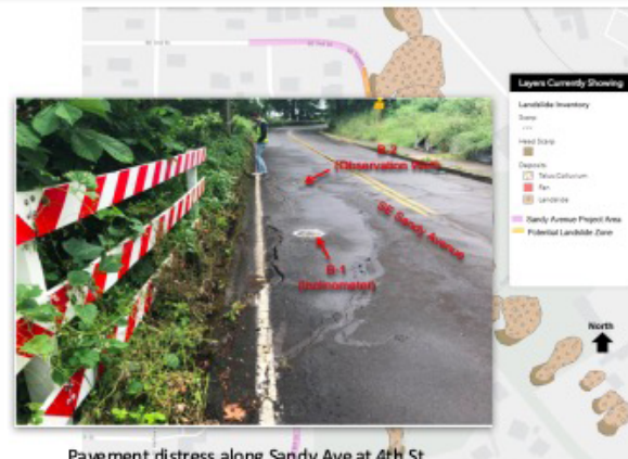
Pavement distress along Sandy Ave at 4th St (Shannon and Wilson, 2018) Landslide hazards along SE Sandy Ave. (DOGAMI, 2018)
