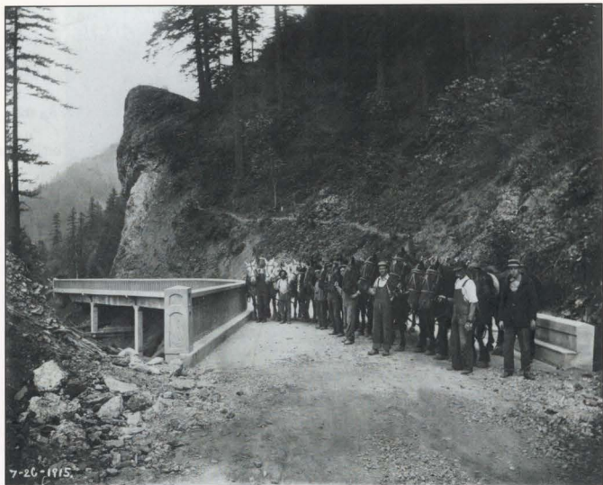
Figure 5. The Building of the Columbia River Highway 1915. Photo Courtesy of ODOT.
