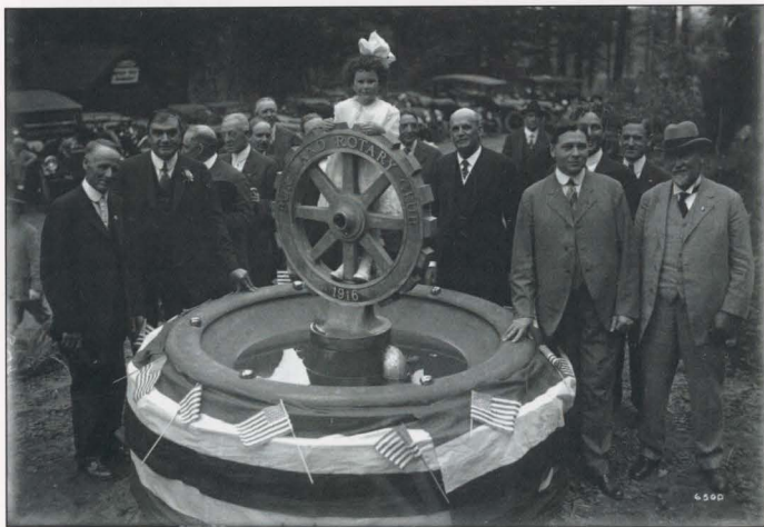
Figure 22. Rotary Club Fountain, Columbia River Highway, at dedication in 1916 (Oregon Historical Society, bb012472).
