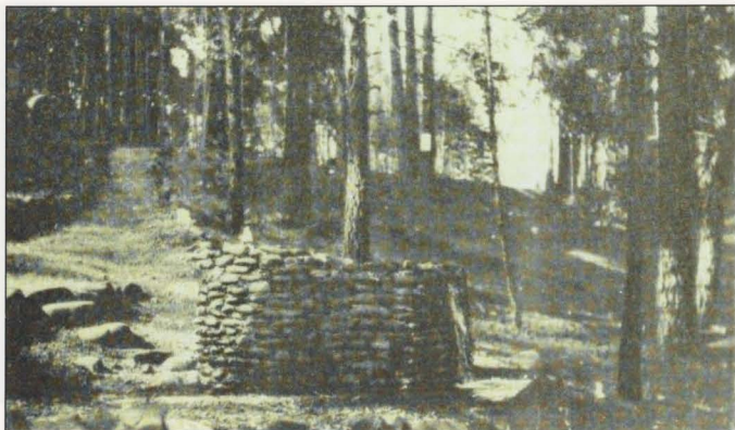
Figure 10. Historic photo of US 199 at the California State Line Fountain, 1930.
