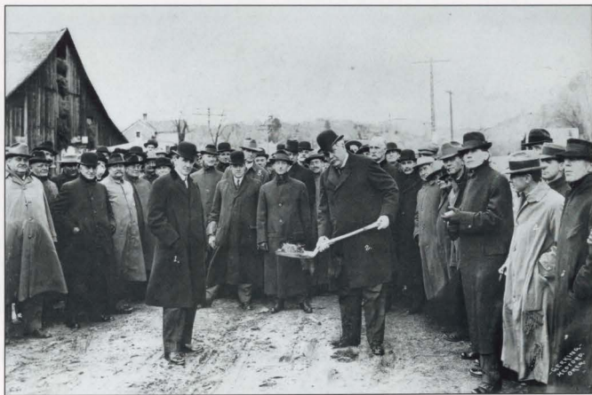
Figure 4. Groundbreaking for the Pacific Highway. Oregon Governor Oswald West and Samuel Hill (with the ceremonial shovel). Jackson County, 1913. Photo courtesy of ODOT.
