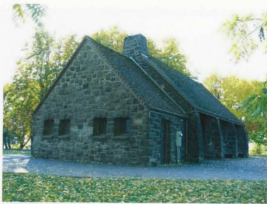
Figure 50: Viewing southwest. Photo by author.
