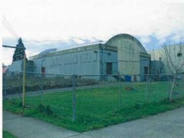
Figure 54: Viewing southwest. Photo by author.
