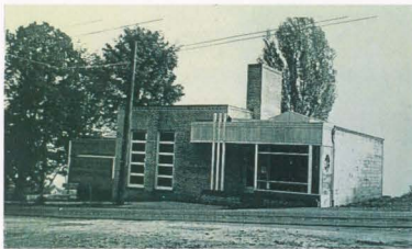
Figure 41: Photo printed in the Works Progress Administration in Oregon, 1938.
