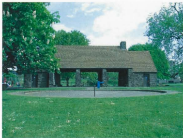
Figure 48: Viewing north. Photo by author.
