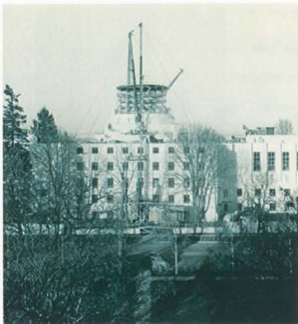
Figure 5: Construction of the Oregon State Capitol by the PWA. Photo courtesy of Oregon State Archives.
