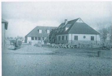
Figure 35: Viewing northeast. Photo courtesy of Oregon Department of Forestry.
