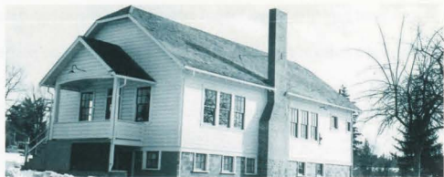
Figure 15: WPA constructed library and community center in Sandy, Oregon. Photo printed in Works Progress Administration in Oregon, 1938.
