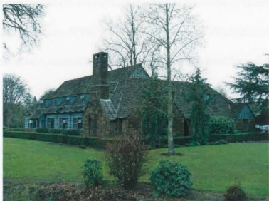
Figure 24: Viewing southwest. Photo by author.
