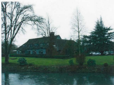
Figure 28: Viewing southwest. Photo by author.
