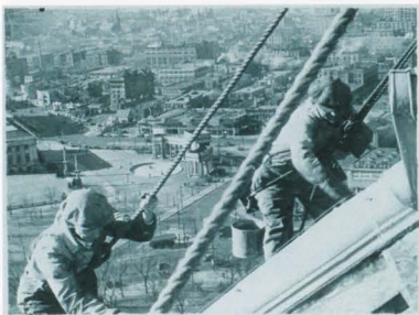
Figure 4: CWA workers cleaning and painting the Denver State Capitol. Photo Courtesy of National Archives and Records Administration.
