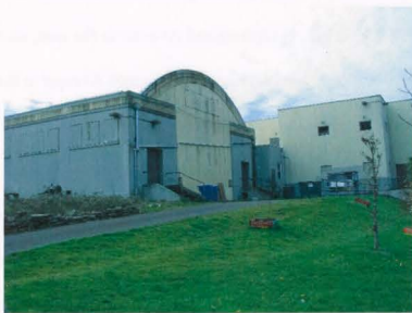
Figure 55: Viewing southwest. Photo by author.
