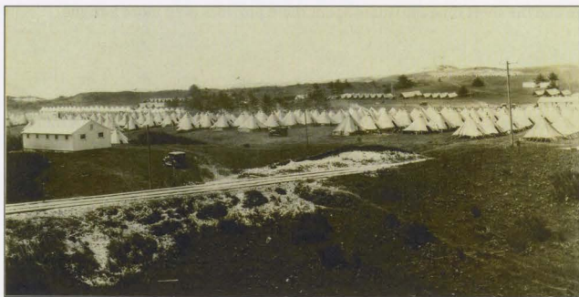
Figure 9: Early construction at Camp Clatsop. Source: Camp Clatsop, c.1915. Photo file 744-F, Oregon Historical Society Research Library.
