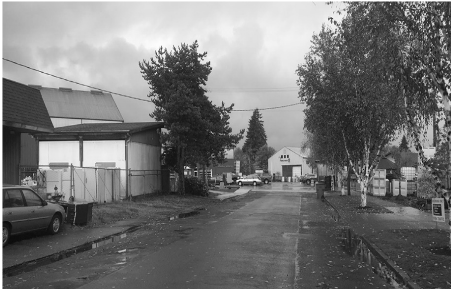
Figure 1: Alpine before renovation.
