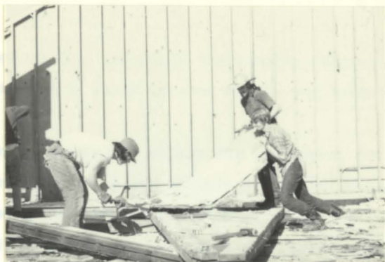
54. Members of a commune disassemble a church in exchange for all salvageable materials.
