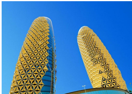
Figure 2: The dynamic solar screen on Al Bahar towers
