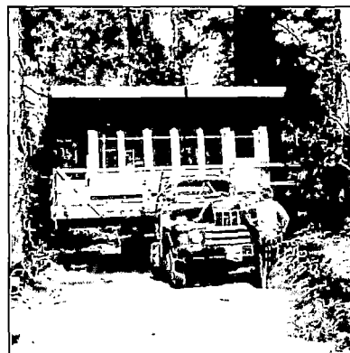
Antelope R-6 lookout preassembled and being transported to the site in 1974 (above). A crane is used to place the R-6 on the tower structure (below). USFS photos.
