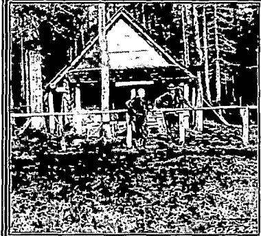
Olallie Meadow cabin constructed in 1910 on Mt. Hood NF in Oregon.
