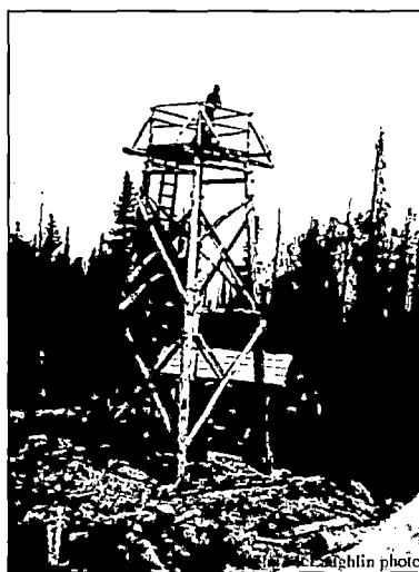
Salmo platform tower on the South side c.1929 with a cabin at the base, Colville NF.
