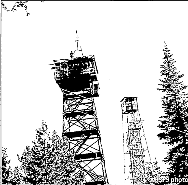
Desolation Butte Lookout construction c.1961
