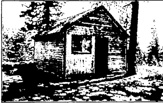
West Myrtle Bunkhouse, building 1017 (1929)
