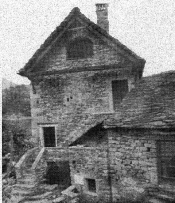
Stone building, Oira, Italy
