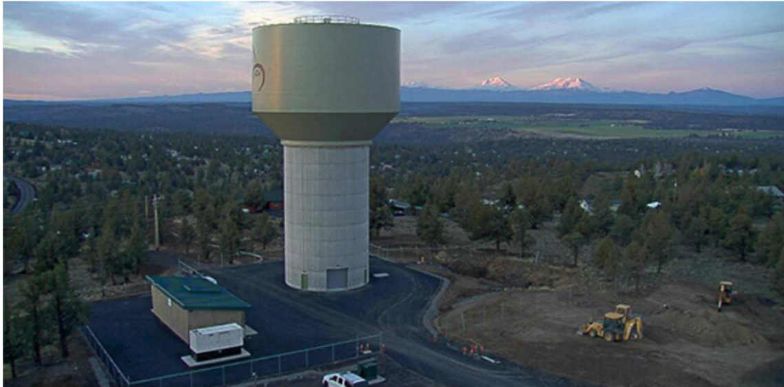
Figure 14. The 700,000 gallon standpipe installed near Crooked River Ranch by Parametrix Services. (Parametrix, Crooked River Ranch Water System Improvements ).
