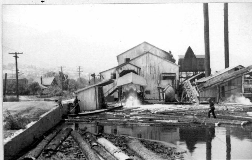
Fig. 44.--Sorting Logs in the Mill Pond.
