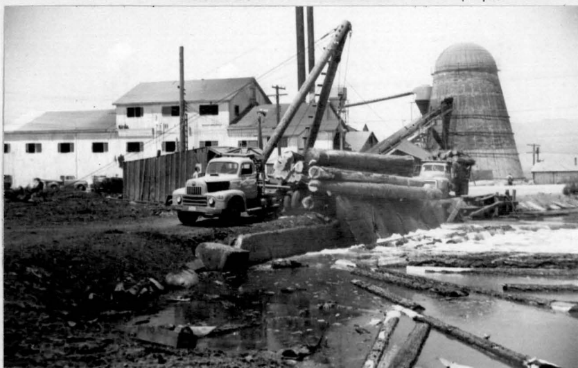
Fig. 43.--Unloading Logs into Mill Pond. Sawmill and waste-burner in background.
