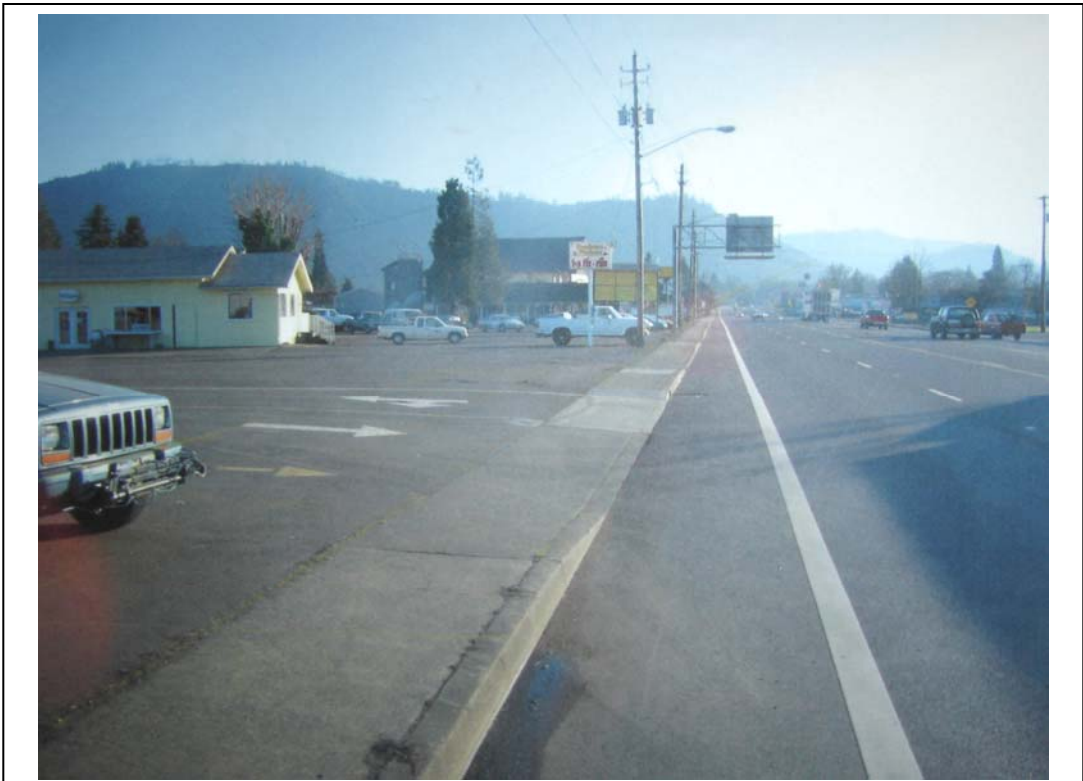
Downtown streetscape, existing
