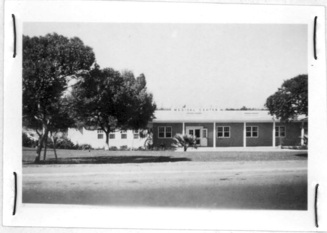
Medical Center Linda Vista Project San Diego
