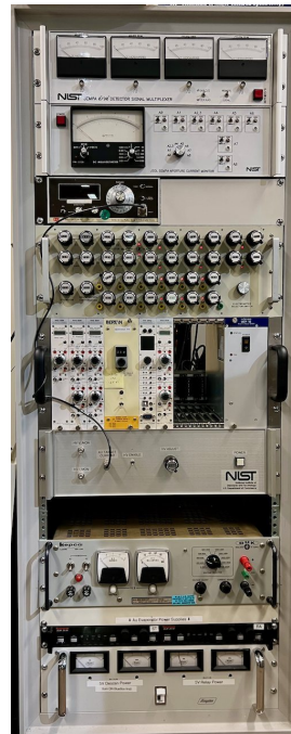
(b) The SEMPA rack on the right
