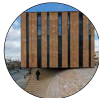
Gallery of Tormeh Office Farhad Mollizadeh Architects
