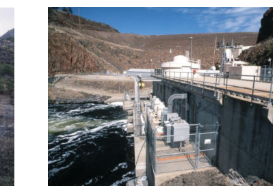
IRON GATE DAM
