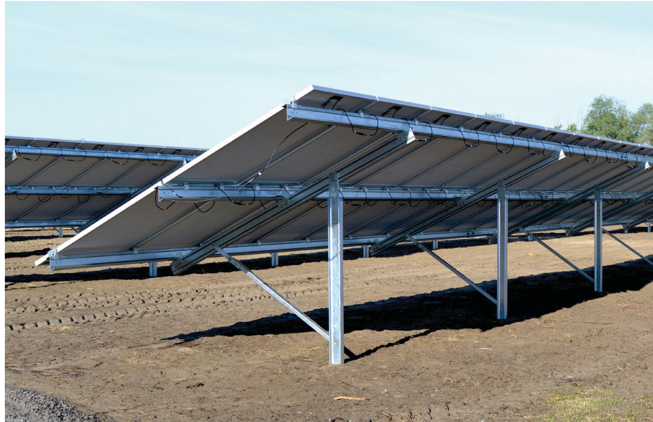
Utility Scale Ground-Mounted P.V. System https://www.solarpowerworldonline.com/2016/11/big-three-avoid-utility-scale-ground-mounting-challenges/
