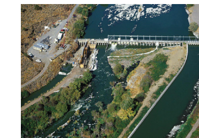
LINK RIVER DAM
