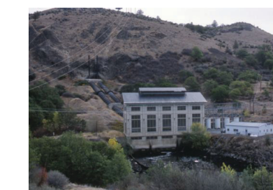
COPCO NO. 2 DAM
