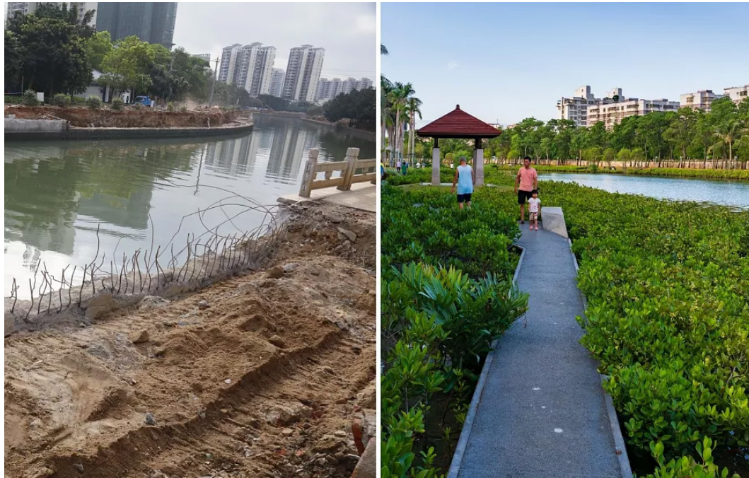
A drainage canal turned stormwater park on the Haikou Meishe River (World Future Council 2016)
