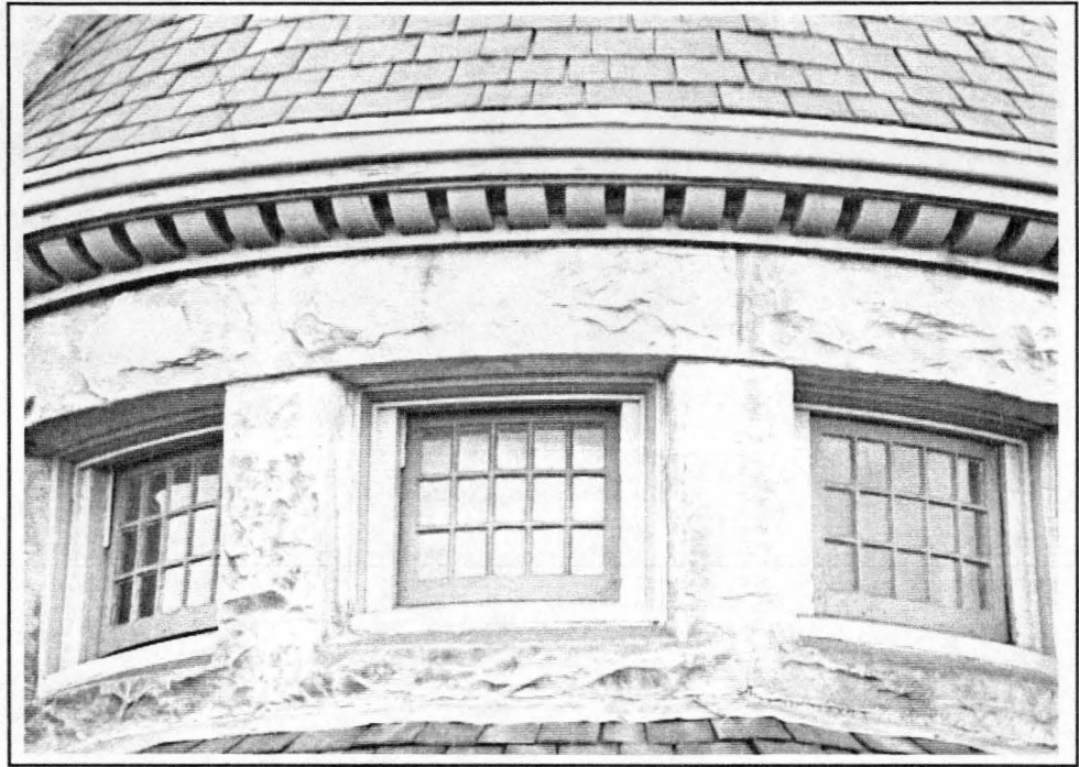
PHOTO 4.27 Upper round tower details, pivotal multi-light windows, dentil course
