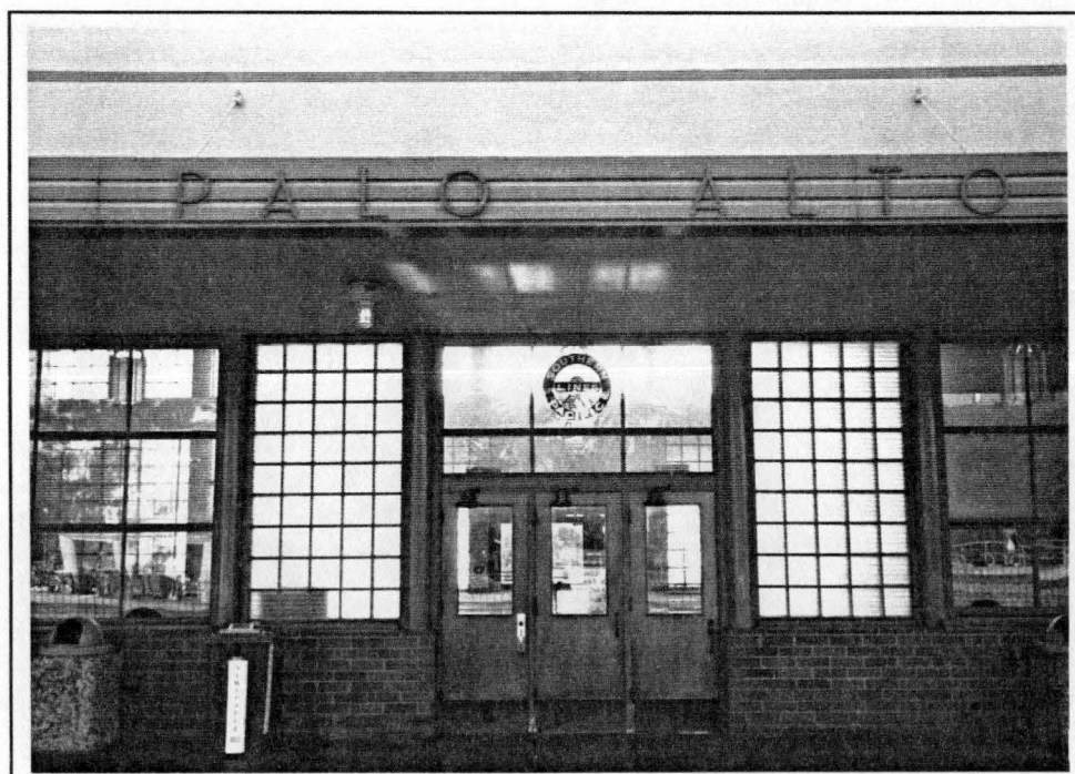
PHOTO 4.66 Trackside entry with Art Deco lettering, glass block sidelights, view of interior space through windows
