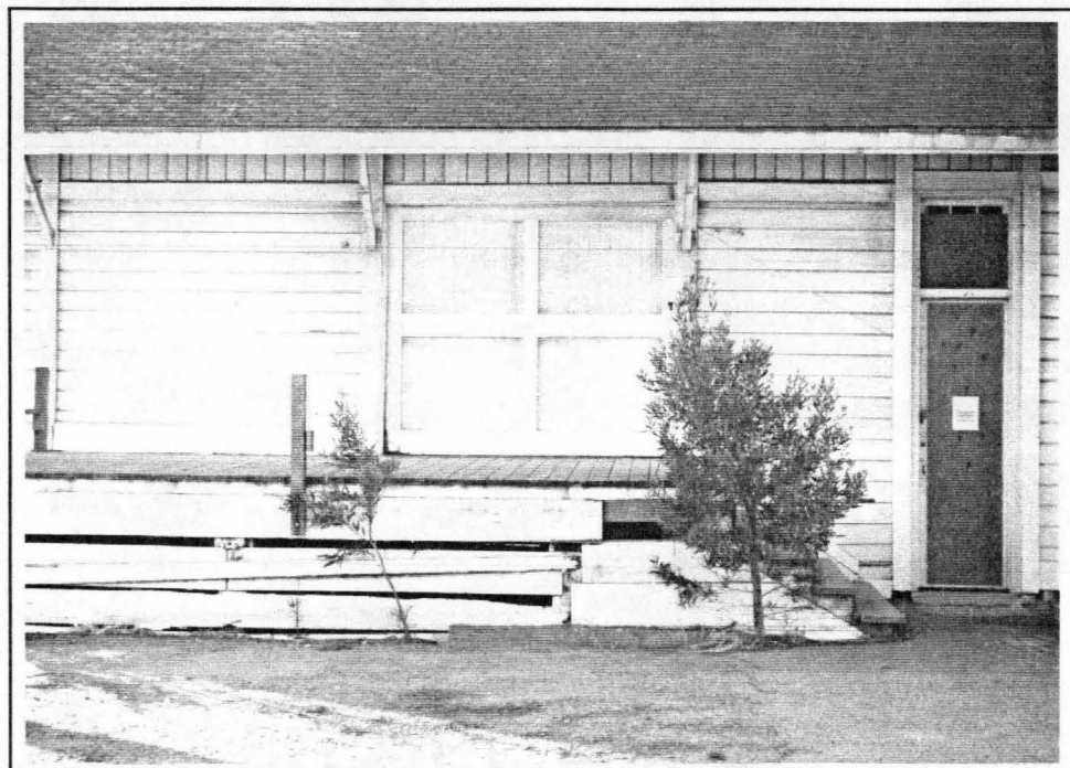
PHOTO 4.14 North trackside loading dock and doors
