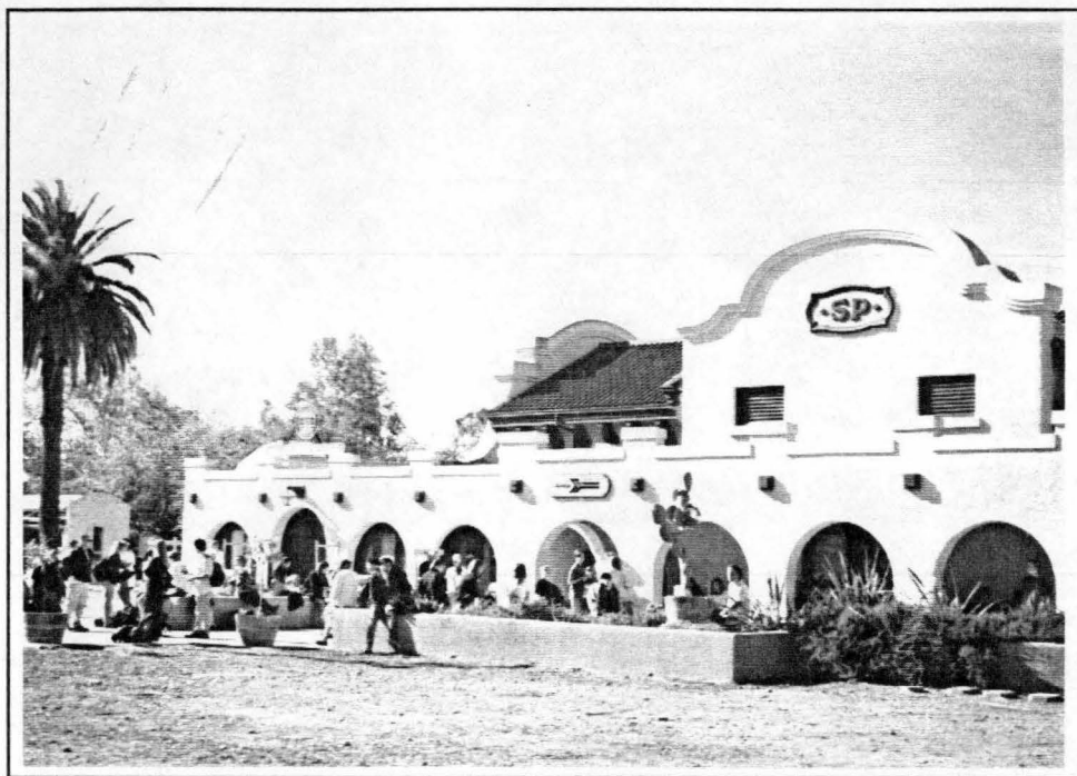
PHOTO 4.37 South trackside view, passengers waiting for the train
