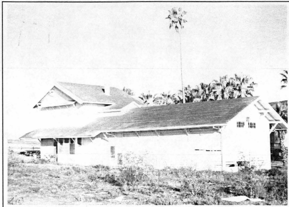
PHOTO 4.10 Benicia Station, combination type, southwest view of front
