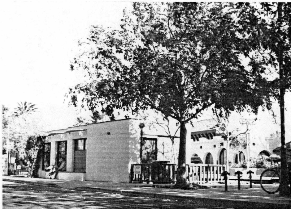
FIGURE 5.6 Compatibly designed bus station at the Davis Railroad Station.
