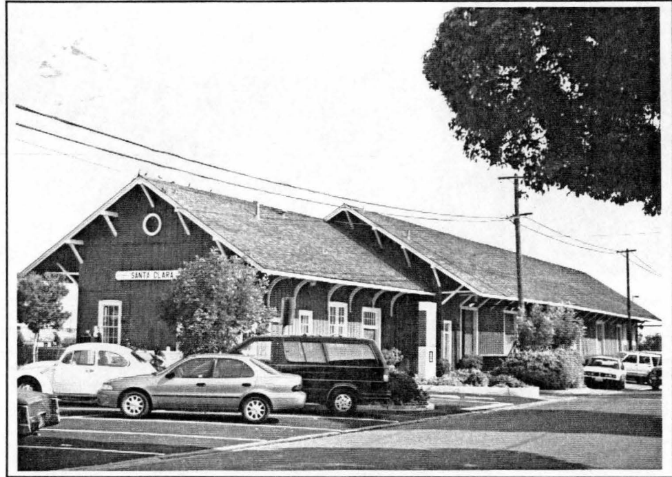
PHOTO 4.1 Santa Clara Station, northwest view, streetside
