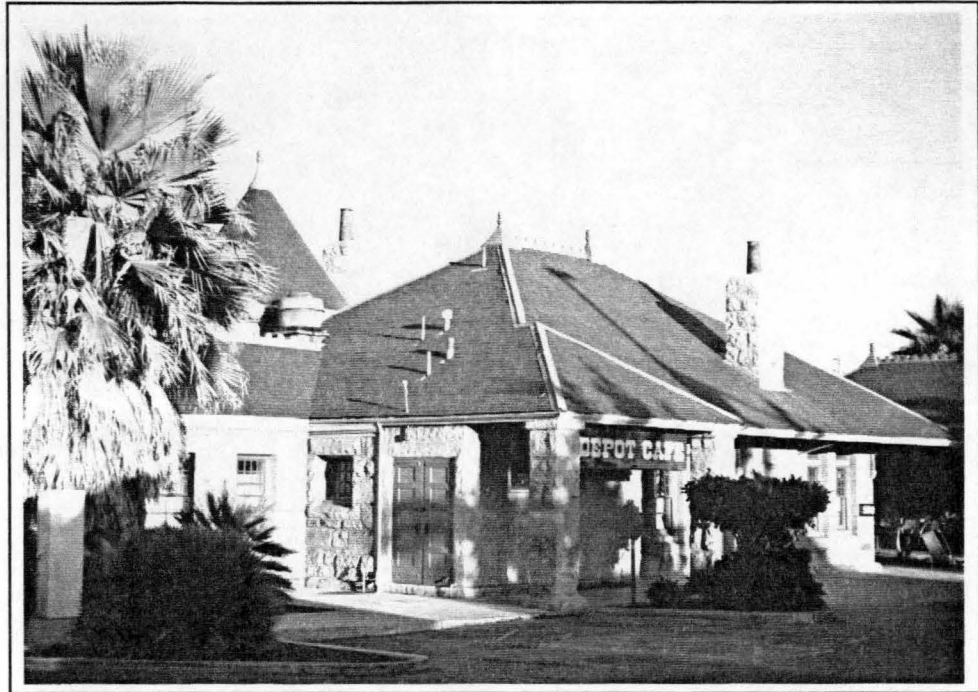
PHOTO 4.25 Partial view of west entry, opposite trackside
