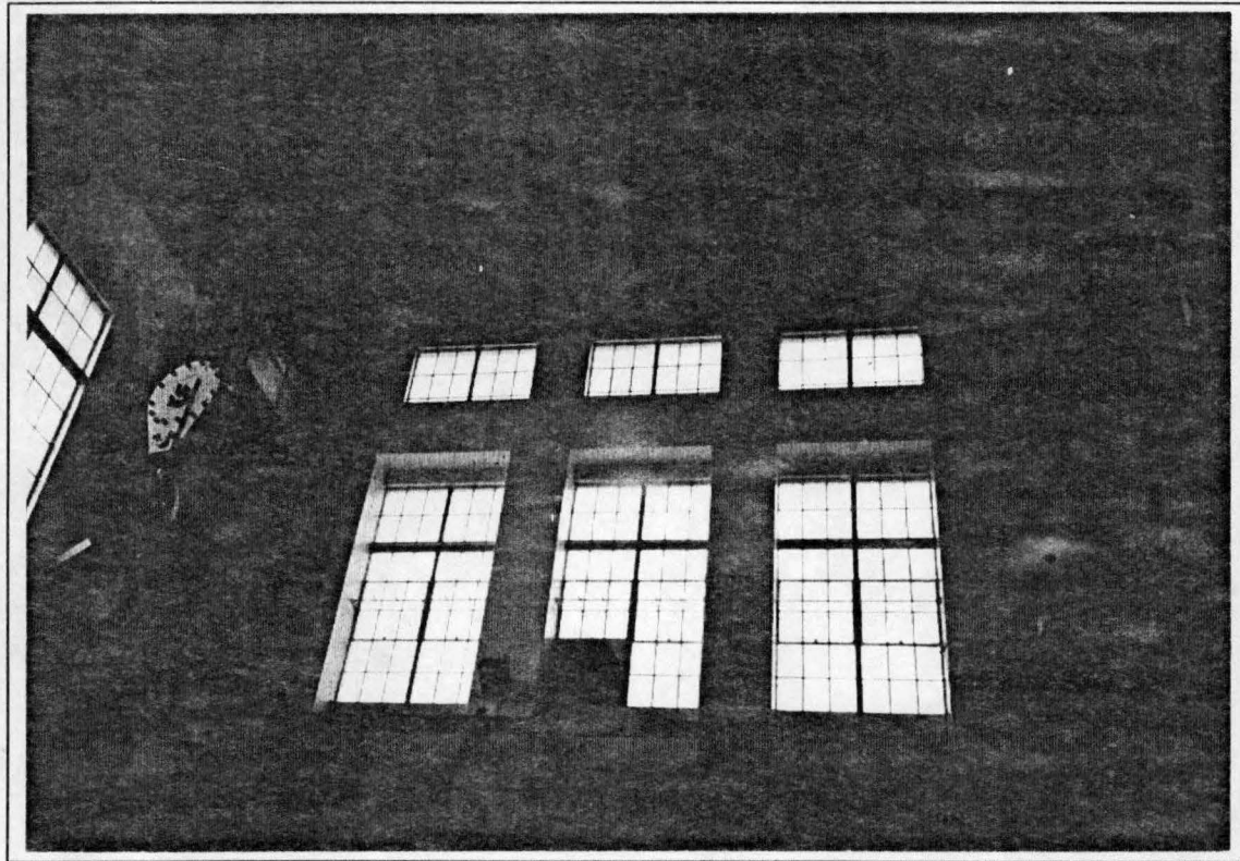
FIGURE 18. Interior of Untanking Tower, Salem Substation, Salem, Oregon.
