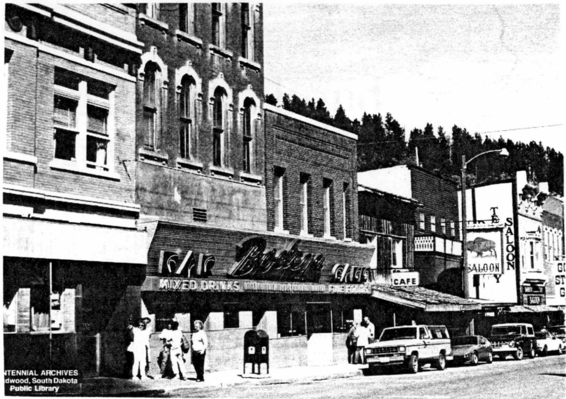
FIGURE 42. The Bodega Bar and Cafe, c. 1987. Long a house of back room gambling, the Bodega, here masked with a "modern" first floor facade from the 1950s or 1960s, was one of the first buildings to undergo a major restoration when gambling was legalized. Source: Centennial Archives, Deadwood Public Library.
