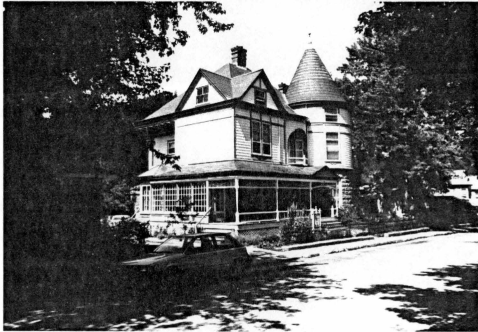
FIGURE 33. The Adams House. Constructed in 1893 for Harris Franklin, the house was purchased by W.E. Adams in the early 1900s. After Adam's death in 1934, his wife went to California. She never returned and the house was unoccupied for over 50 years. When the house was purchased in the 1988, the new owners discovered that the contents of the mansion were just as Mary had left them, including the linens on the beds, magazines from the week she left, sympathy cards from Adam's funeral, silver in the wall safe, china in the cabinet, and rock-hard cookies in the pantry. The house has undergone minor repairs and maintenance, but remains essentially unchanged from the 1930s and is used as a Bed and Breakfast Inn. Photo by author, 1993.
