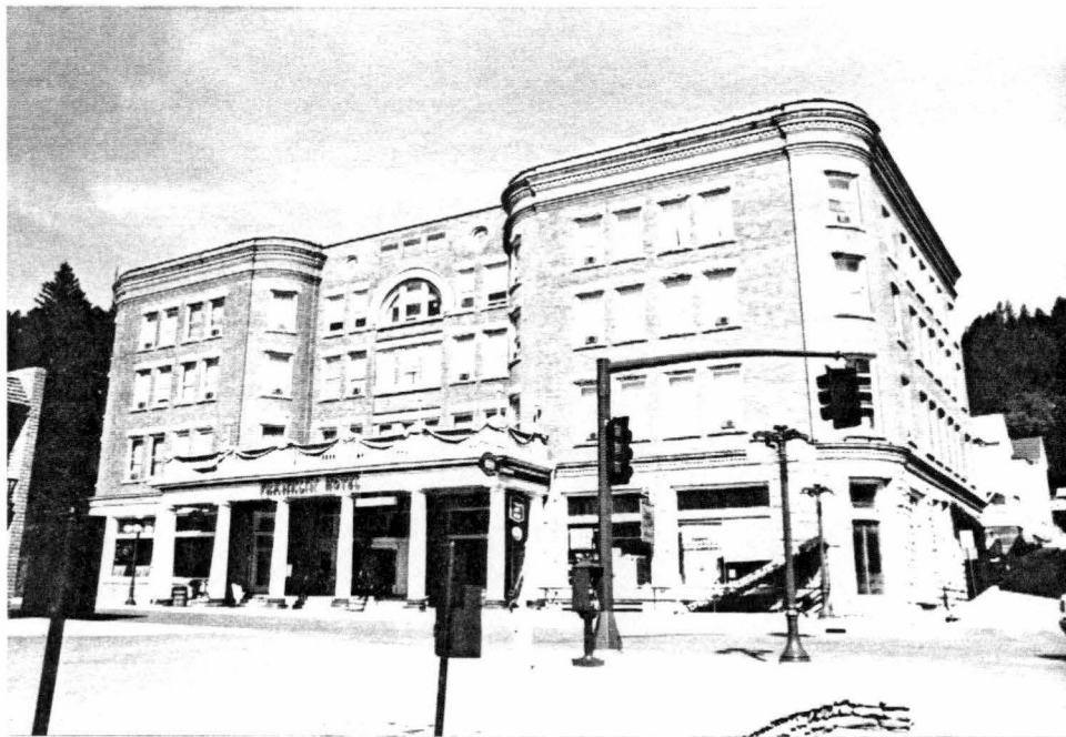
FIGURE 38. The Franklin Hotel in 1993. Restoration work at the time this photograph was taken was limited primarily to interior work. The porch and balcony has been repaired, but the cornice on the center portion of the building is still missing. Photos by author, 1993.
