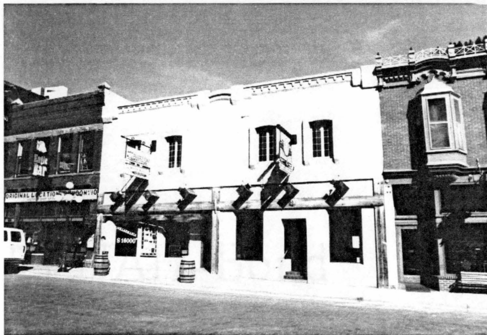
FIGURE 57. Prairie Edge Gaming. An example of inappropriate renovation of an old building made to look like an adobe structure, complete with vigas, from the southwest. Photo by author, 1993.
